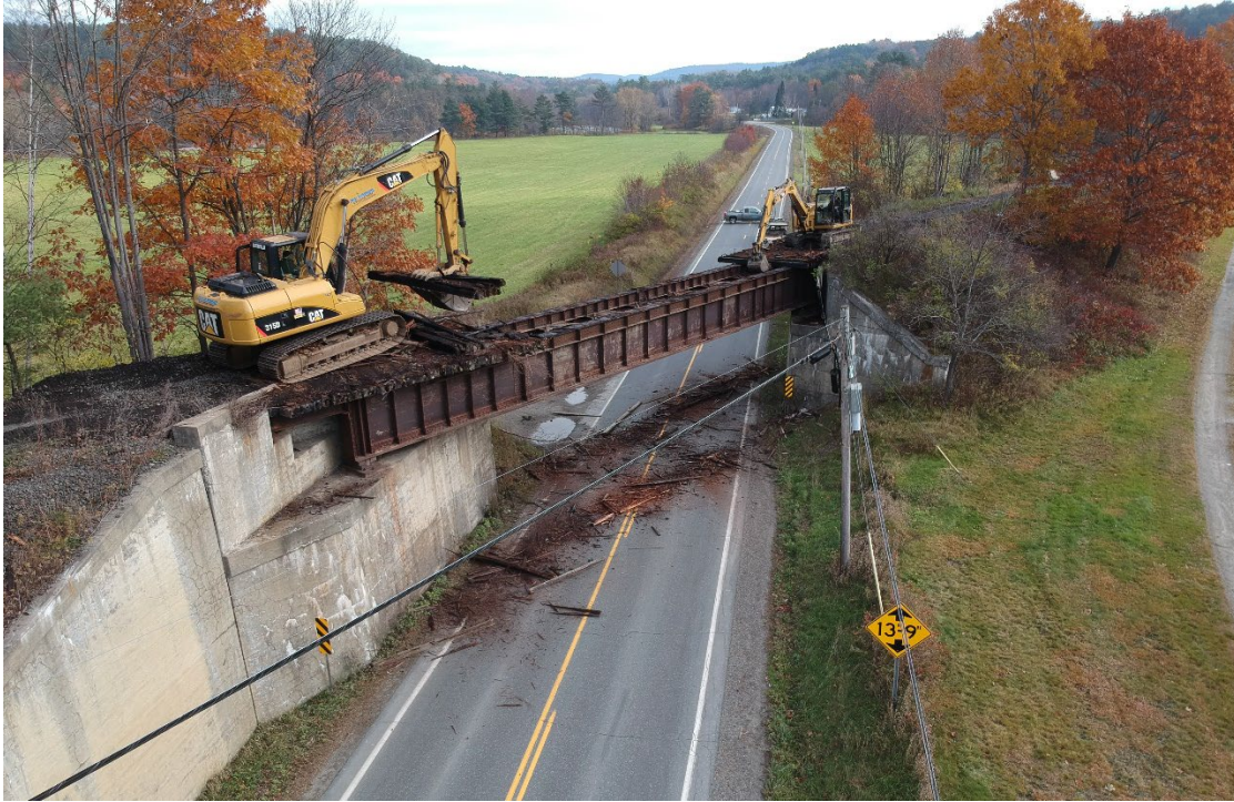
Replacing a bridge deck on the Ammonoosuc Rail Trail in Haverhill.
