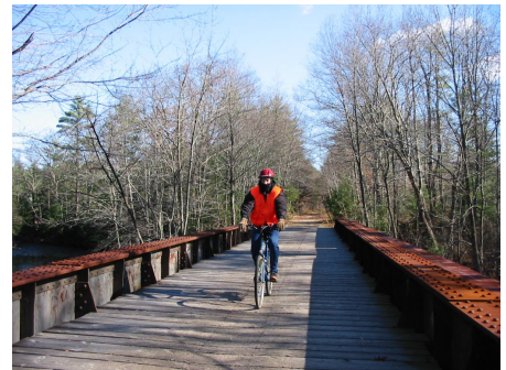
Rail Bridge over Lamprey River
