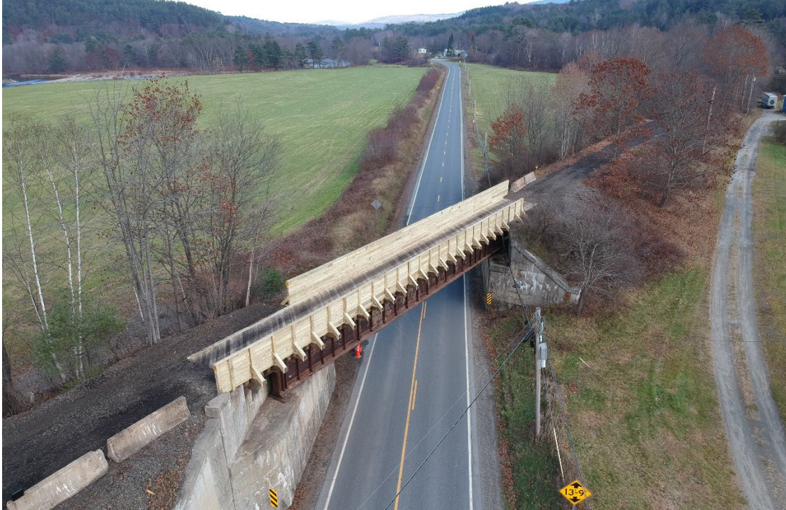
The finished bridge deck on the Ammonoosuc Rail Trail in Haverhill.
