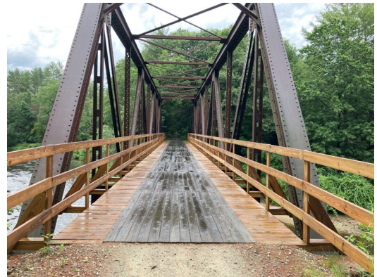
Sugar River Truss Bridge
