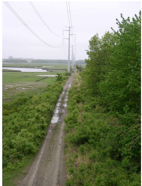
Hampton Branch corridor through wetlands as seen from Route 1
