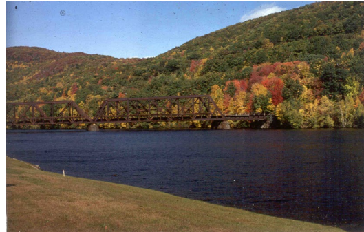
Rail bridge over Connecticut River
