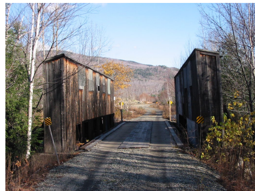
Boxed Pony Truss Bridge on Rail Trail
