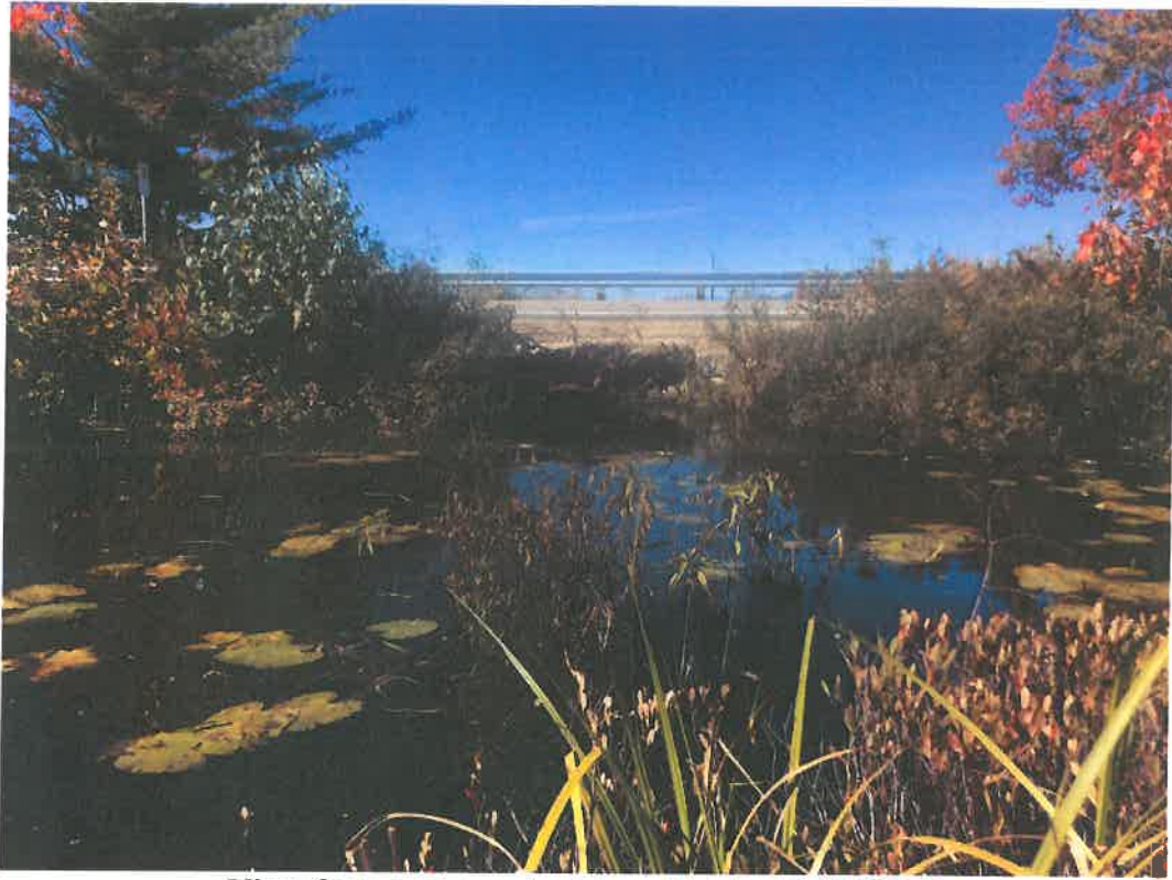
View from upstream looking at inlet – 10/17/2018
