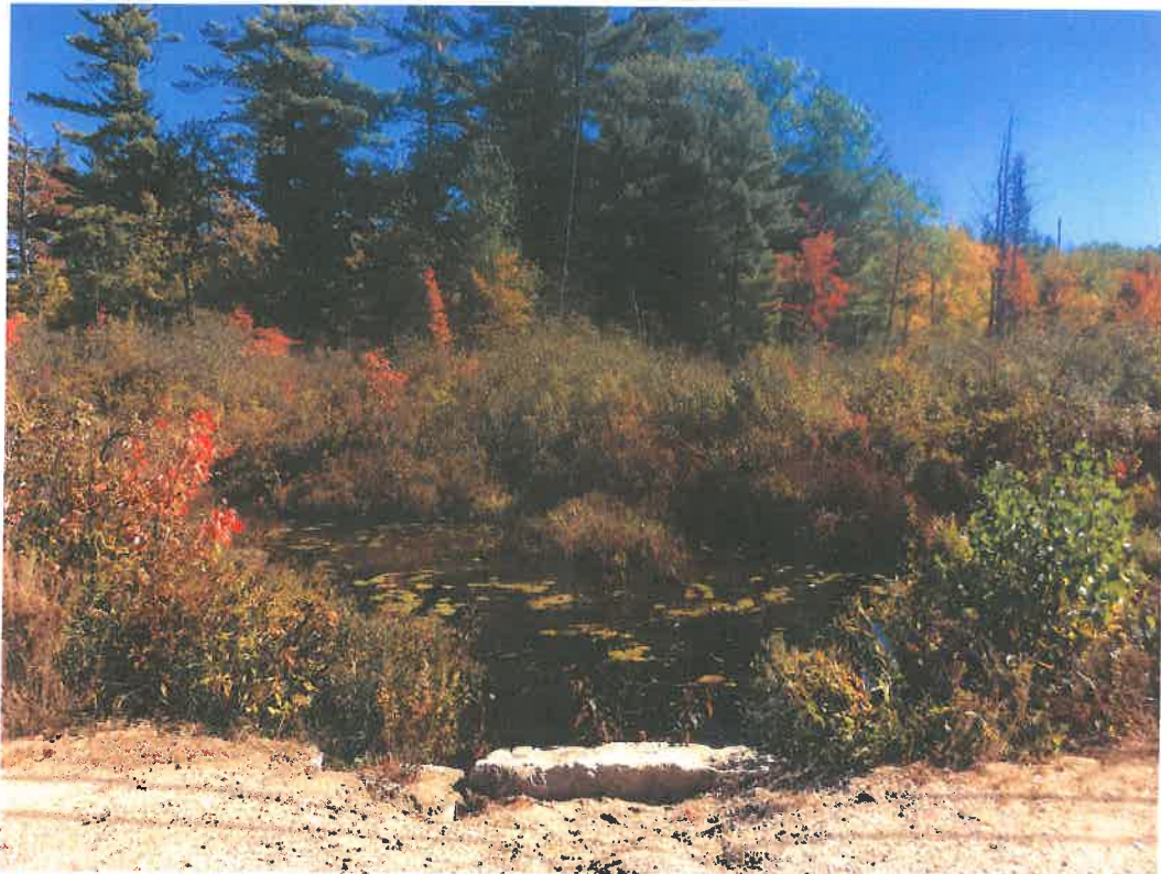
View of Inlet from roadway – 10/17/2018
