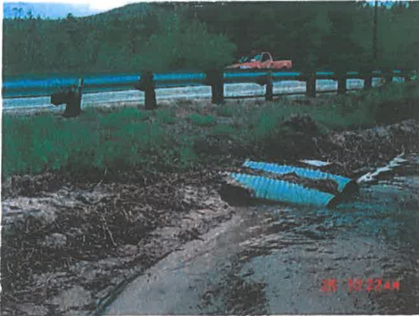
Outlet end (Looking southeast)
