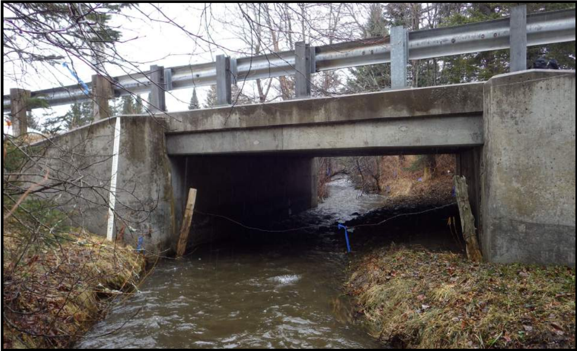
Photo 3: Inlet looking downstream
