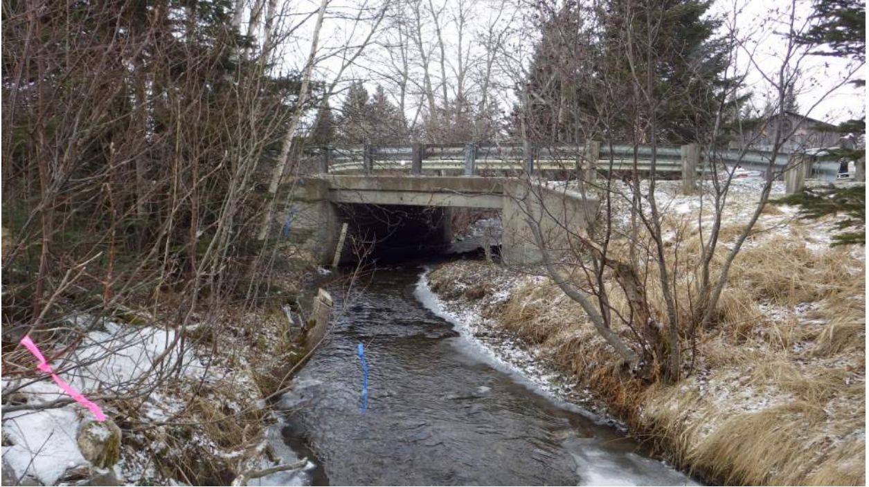
Inlet side looking downstream
