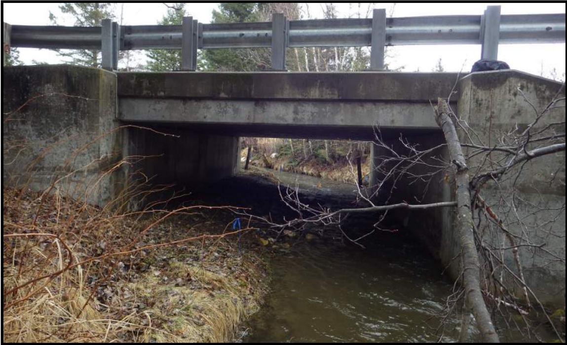
Photo 1: Outlet looking upstream
