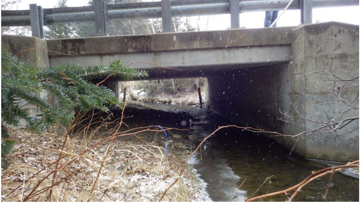
Through structure downstream looking upstream
