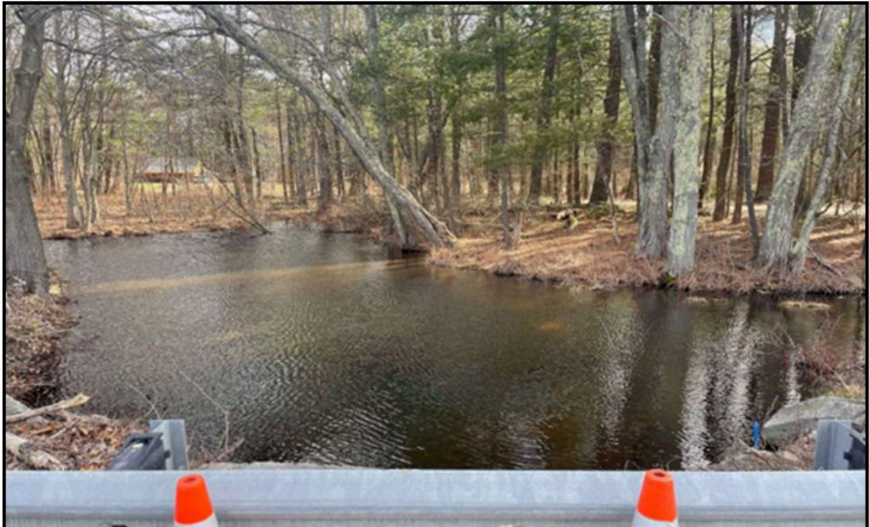
Photo 8: Upstream channel from Culvert (4/7/23) R. Thomson
