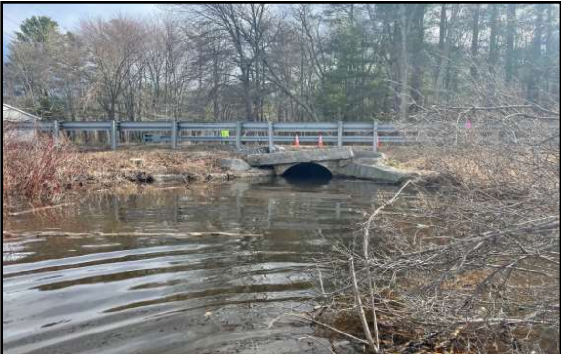
Photo 2: Outlet looking east toward structure.
