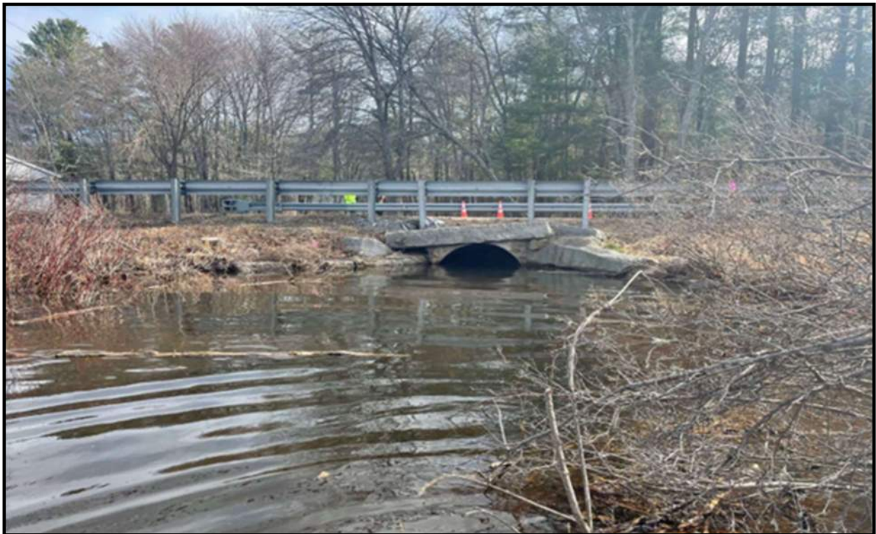
Photo 2: Culvert Outlet from Massabesic Lake (4/7/23) R. Thomson
