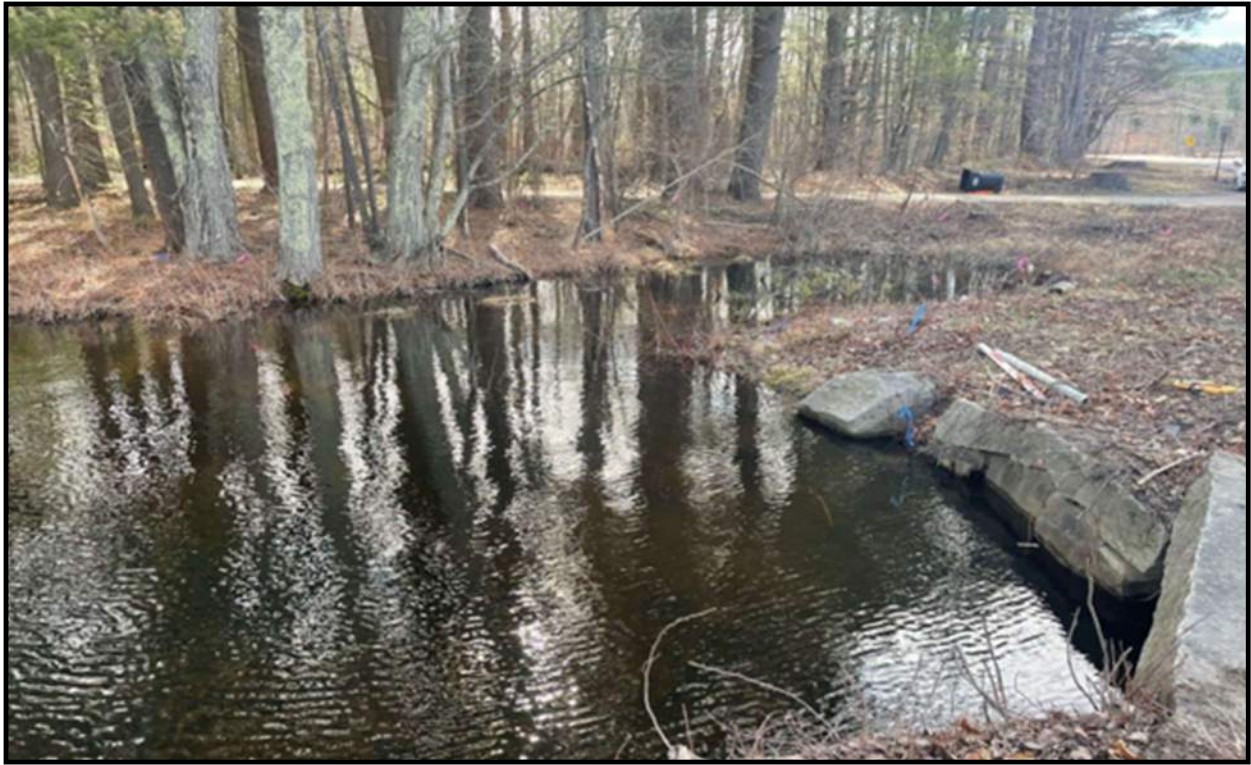
Photo 7: From Culvert inlet looking upstream towards right bank (4/7/23) R. Thomson
