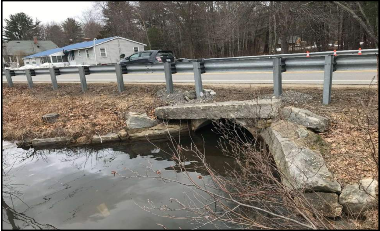
Photo 1: Culvert Outlet (3/24/23) J. Commerford
