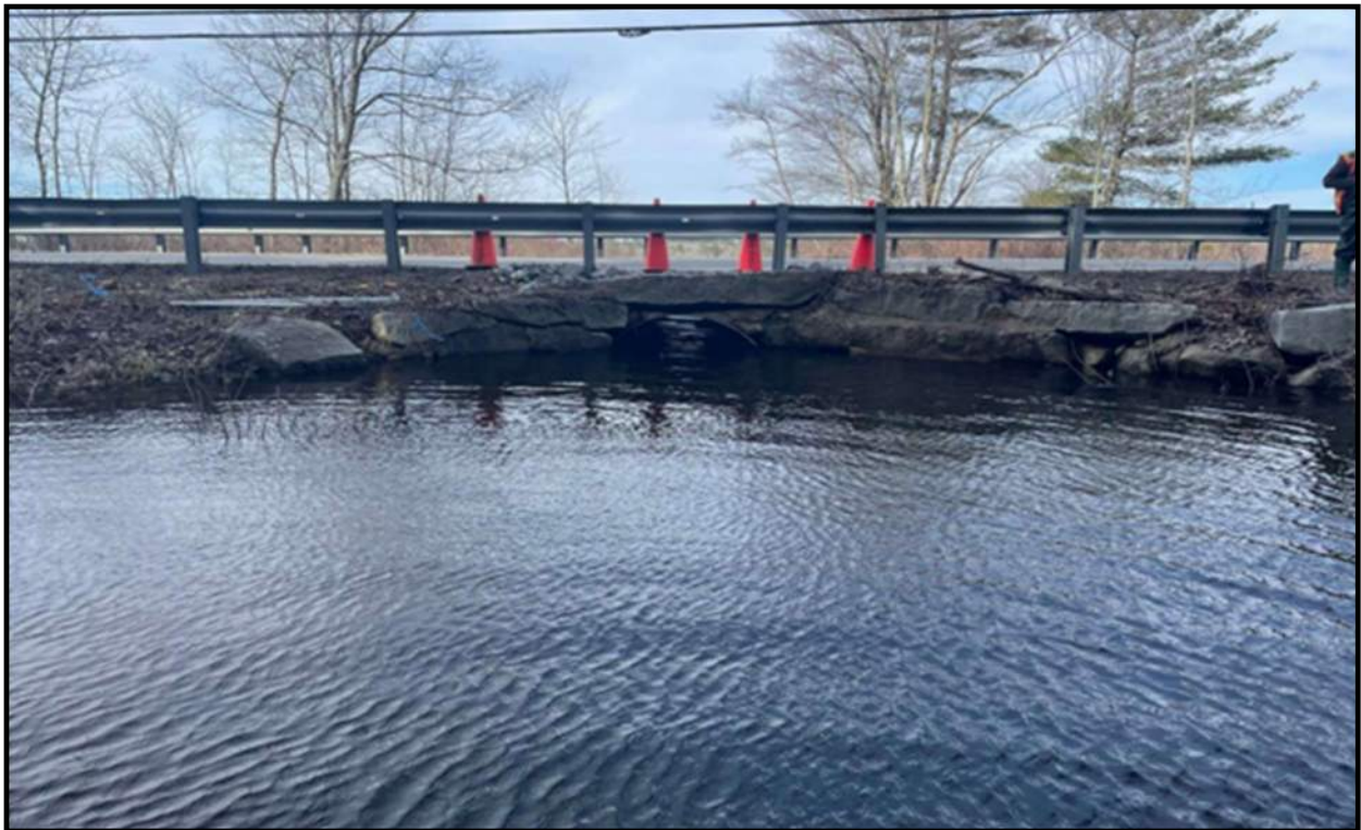
Photo 6: Looking at the Culvert Inlet from Upstream (4/7/23) R. Thomson
