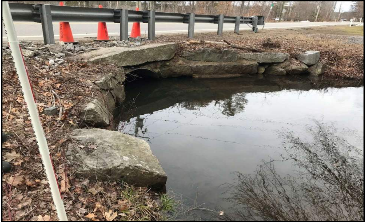
Photo 5: Culvert Inlet (3/24/23) J. Commerford
