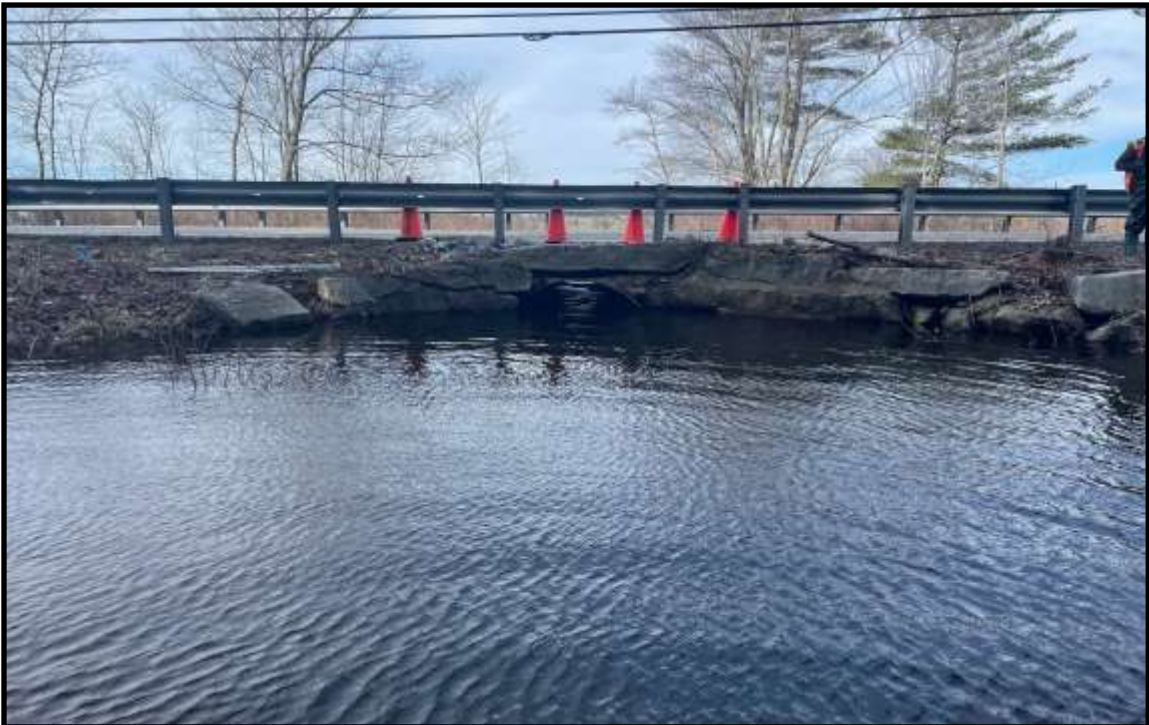
Photo 4: Inlet looking west downstream at structure.
