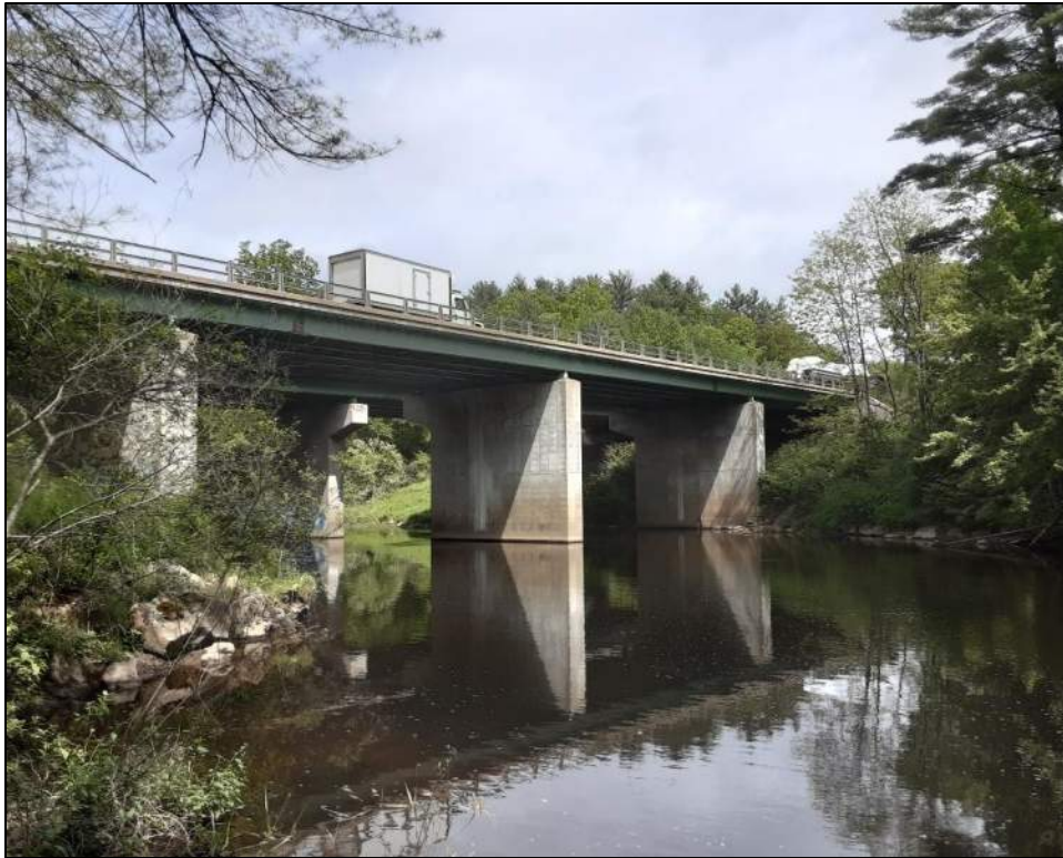
Photo 3. View northwest of Bridge No. 106/133 (Northbound) Photo taken 5/27/22
