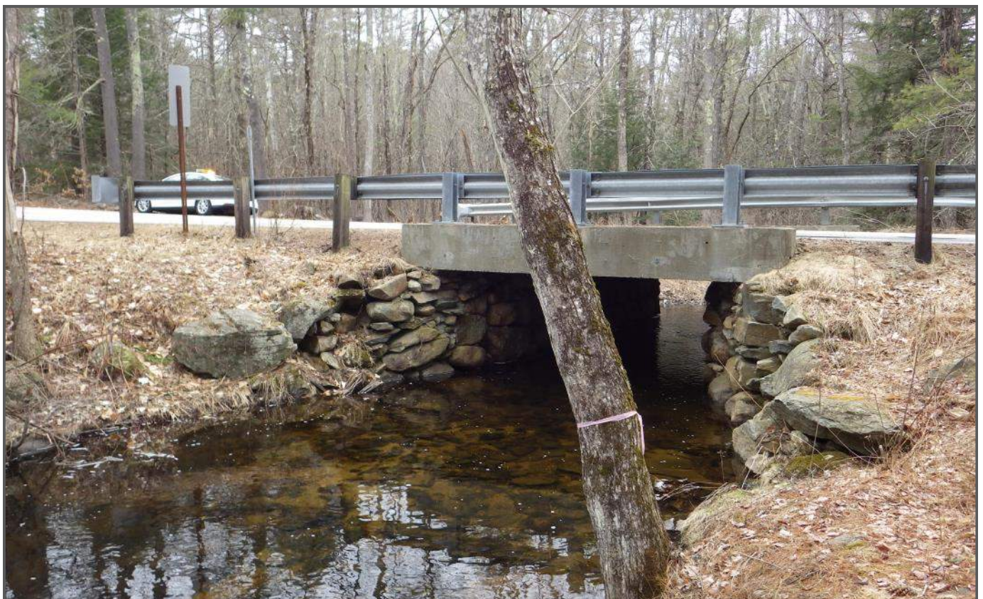
Photo 8: Looking Northwest (Upstream) at Outlet
