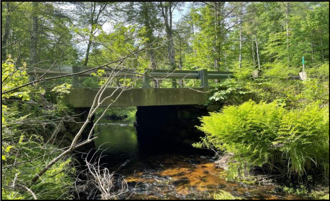
Photo 3: Inlet looking downstream
