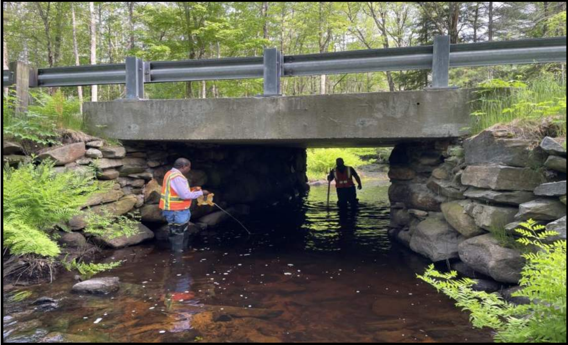
Photo 1: Outlet looking upstream
