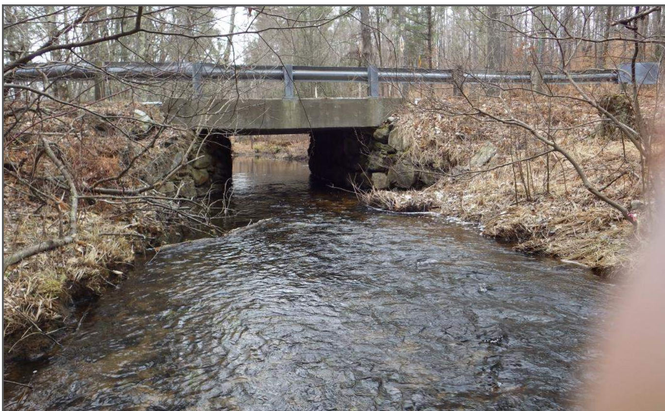
Photo 4: Looking Southeast (Downstream) at Inlet
