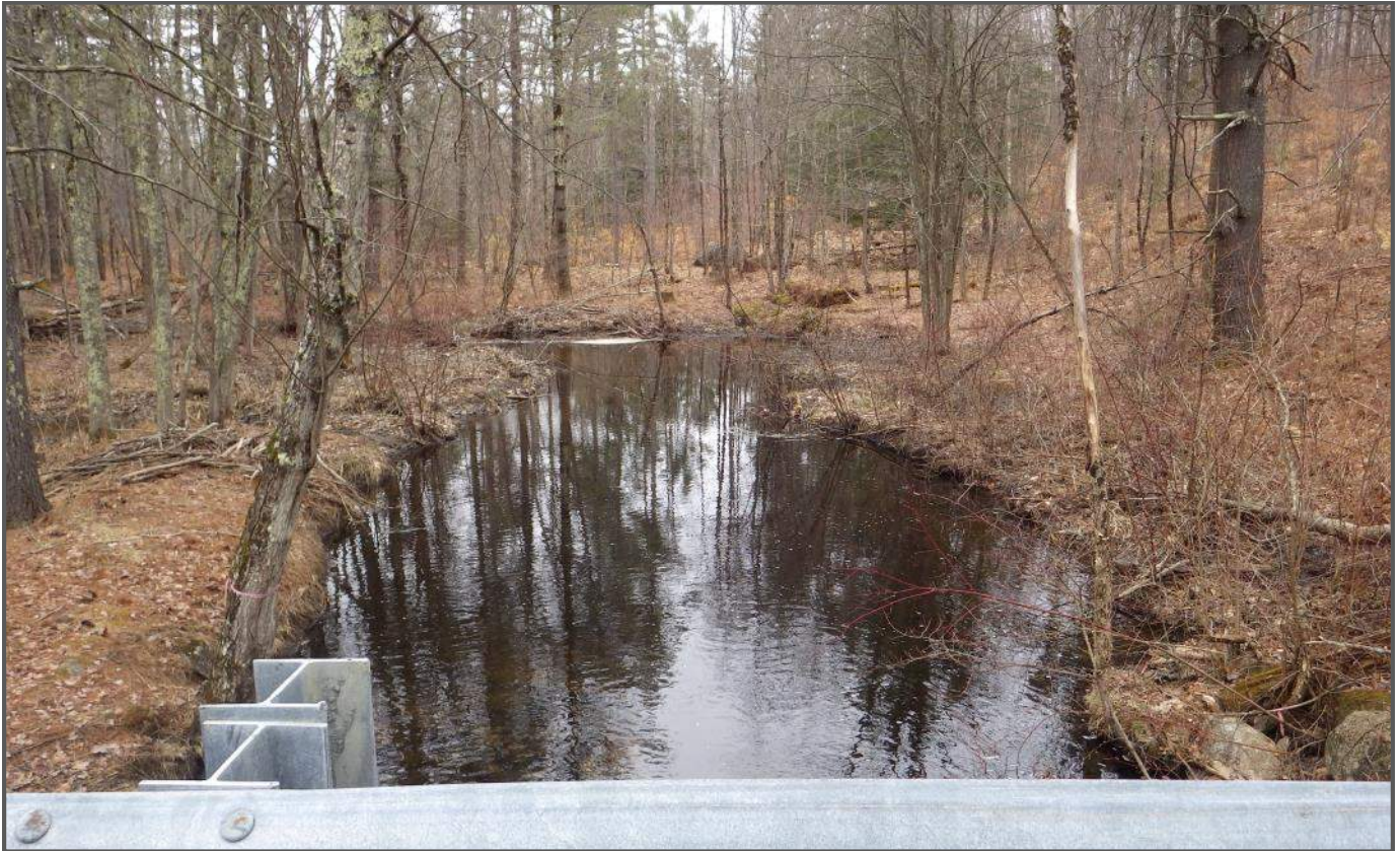
Photo 7: Looking Southeast (Downstream) From NH 136
