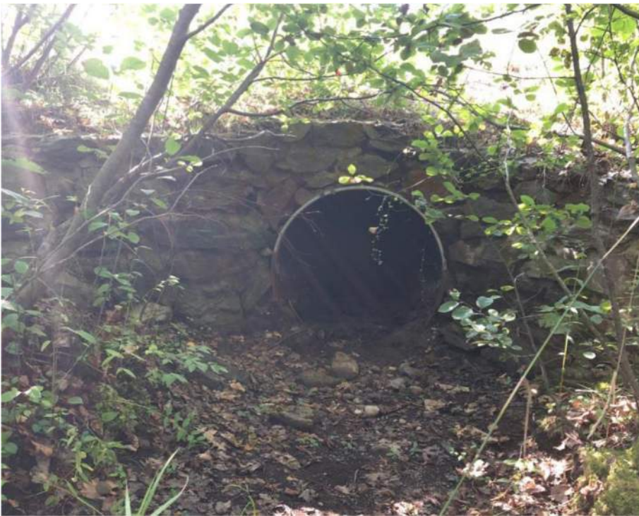
8. Facing culvert 24121 (inlet)
