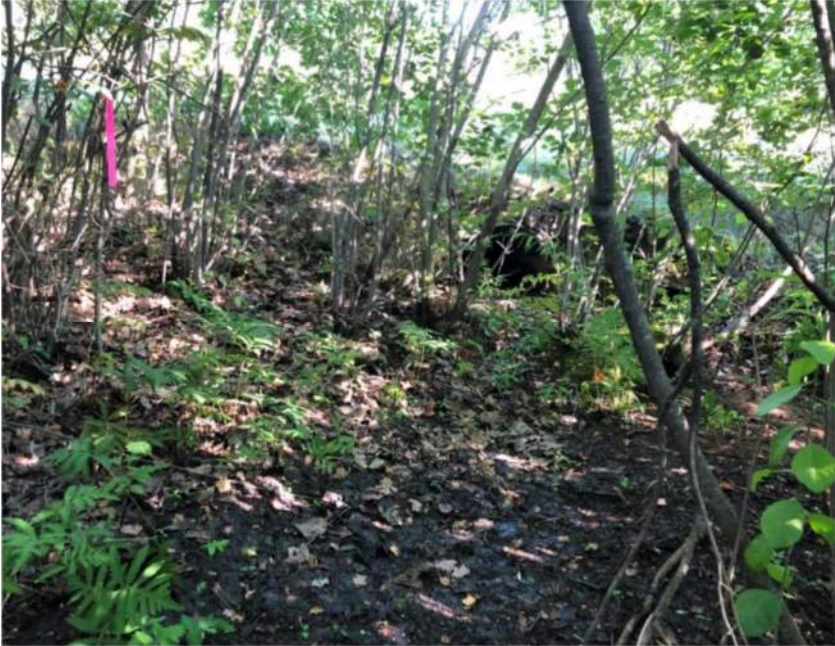
7. Facing culvert 24121 impact area (outlet)
