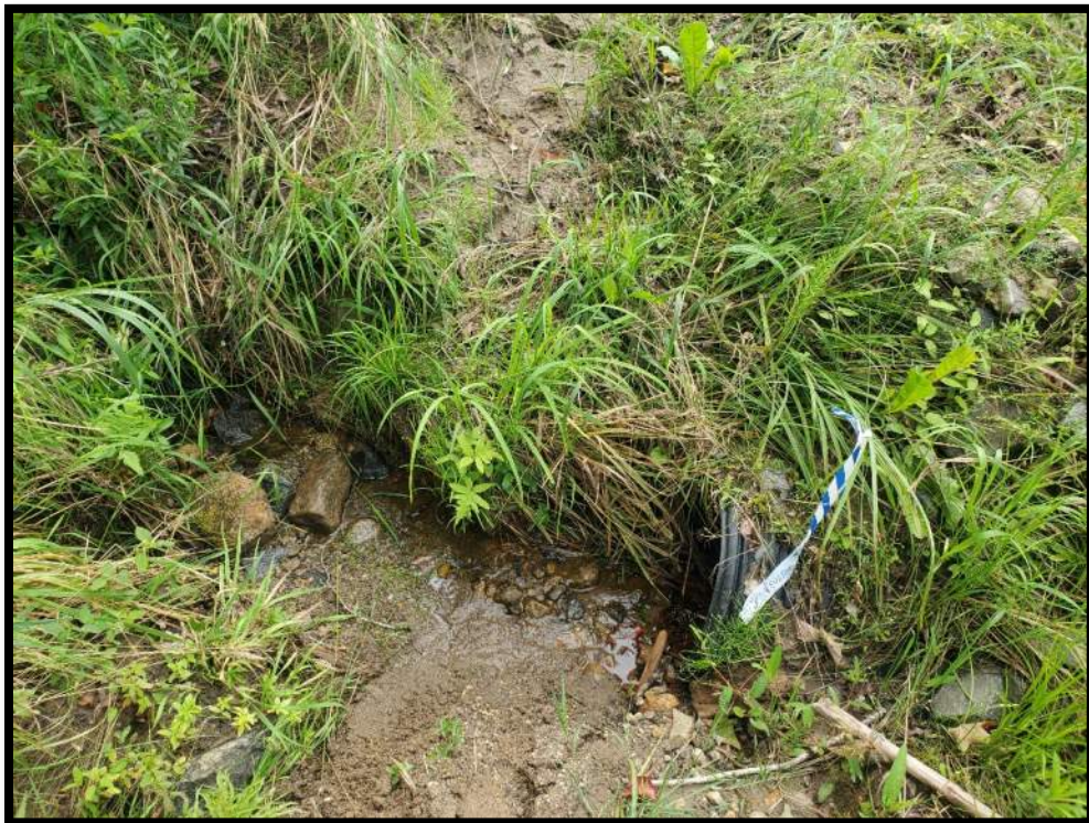
Photo 8 – Stream 3 View of Culvert Inlet – 8/14/2023
