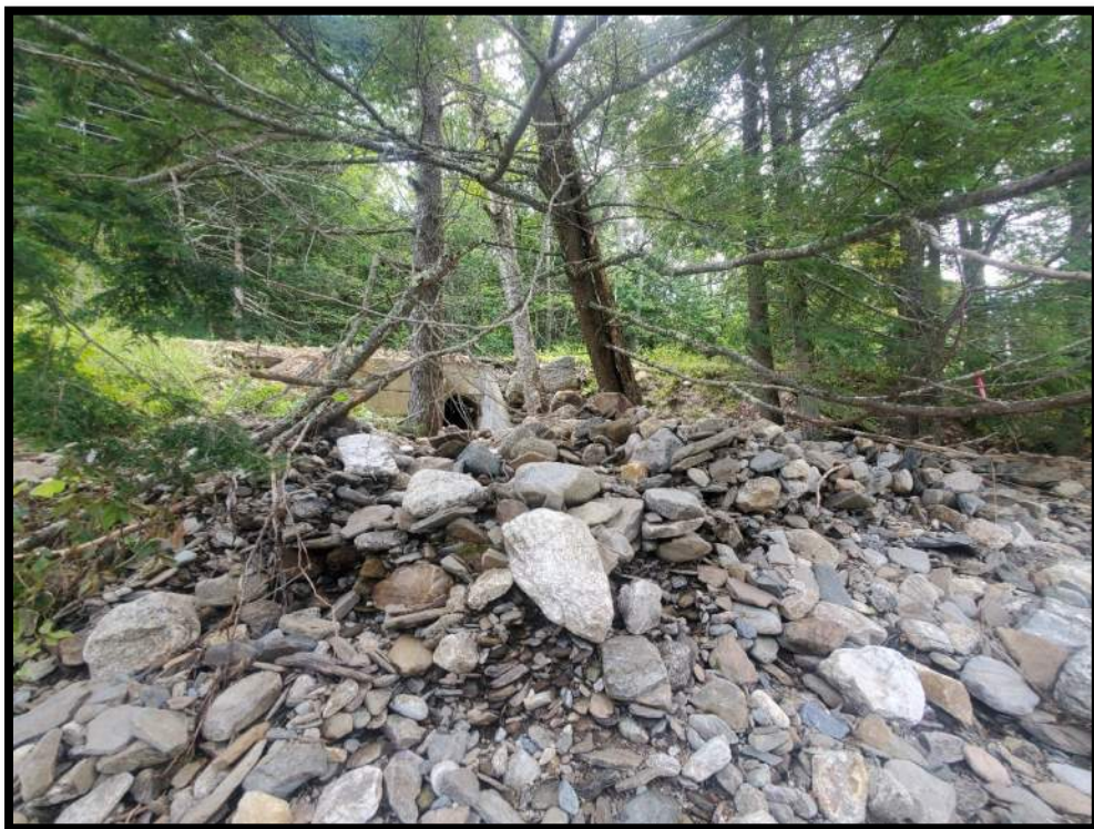
Photo 4 – Stream 1 View of Culvert Outlet Facing Southeast – 8/14/2023
