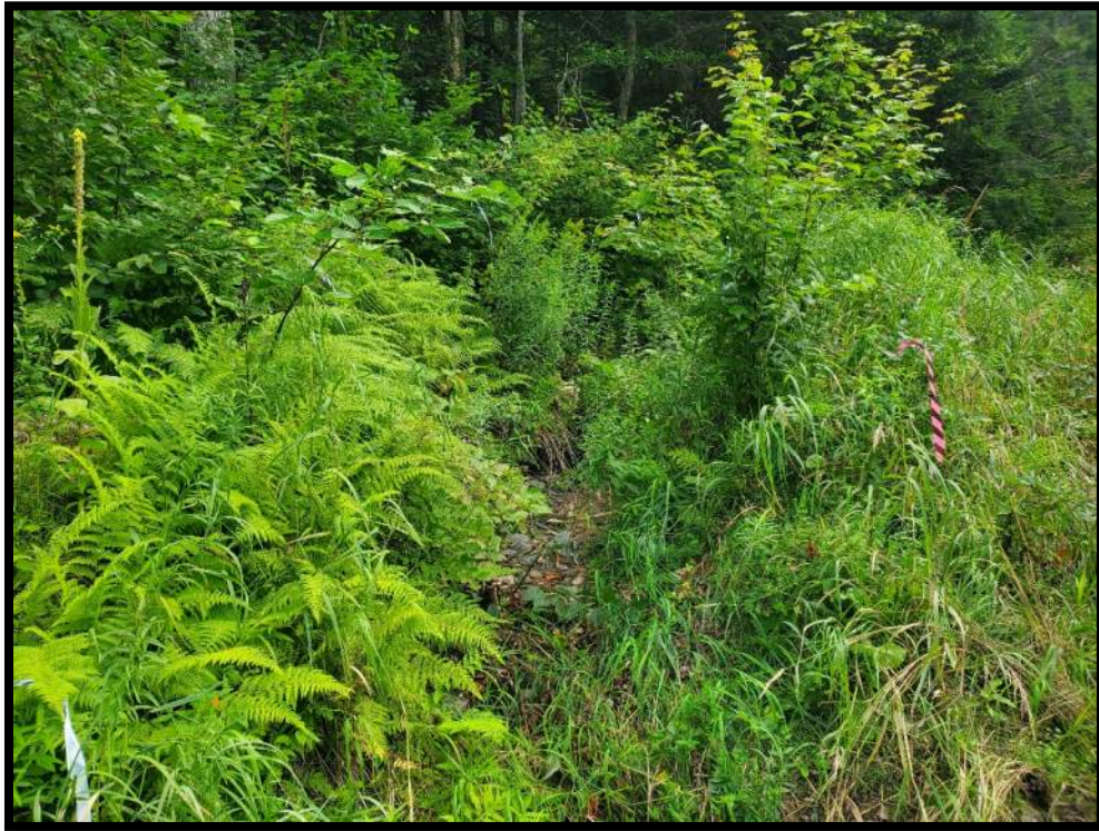
Photo 7 – Stream 3 View from Culvert Inlet Facing Upstream – 8/14/2023
