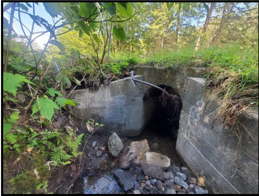
Photo 3 – Stream 1 Inlet Facing Downstream – 8/14/2023
