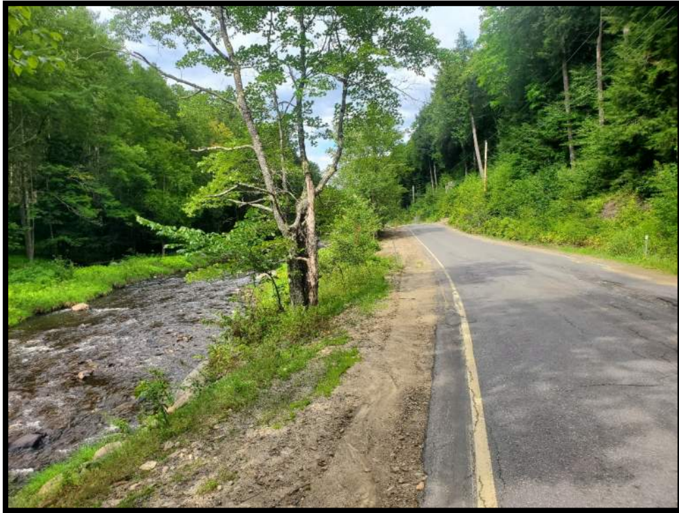
Photo 1 – View of Route 123A and Cold River from West Edge of Project Facing East – 8/14/2023
