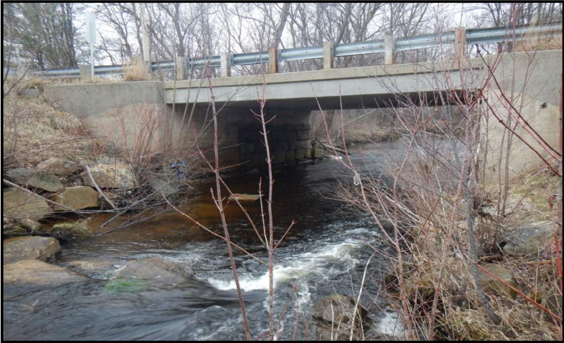
Photo 3: Inlet looking downstream
