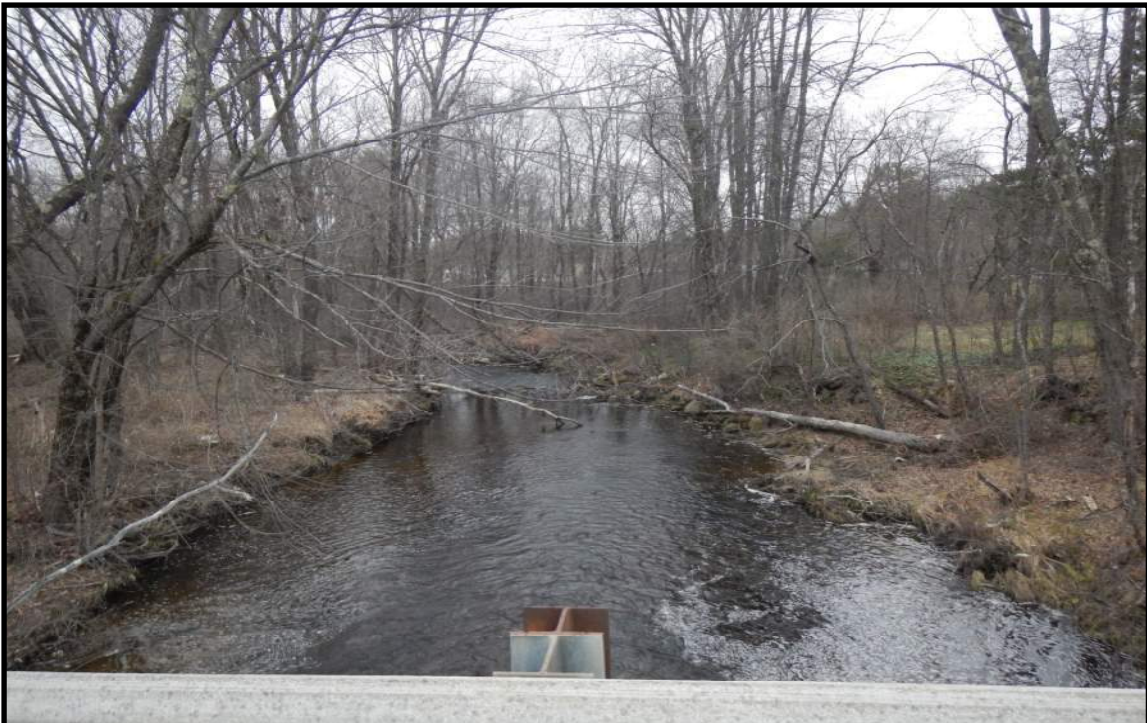
Photo 2: Outlet looking downstream
