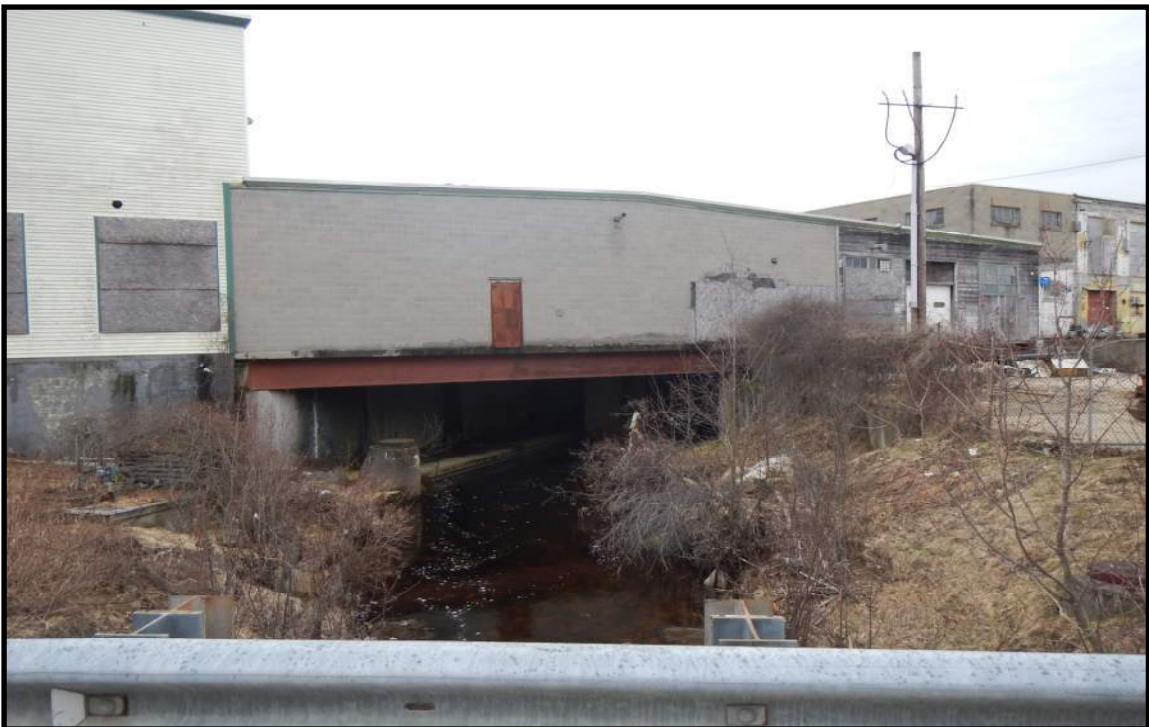
Photo 4: Inlet looking upstream
