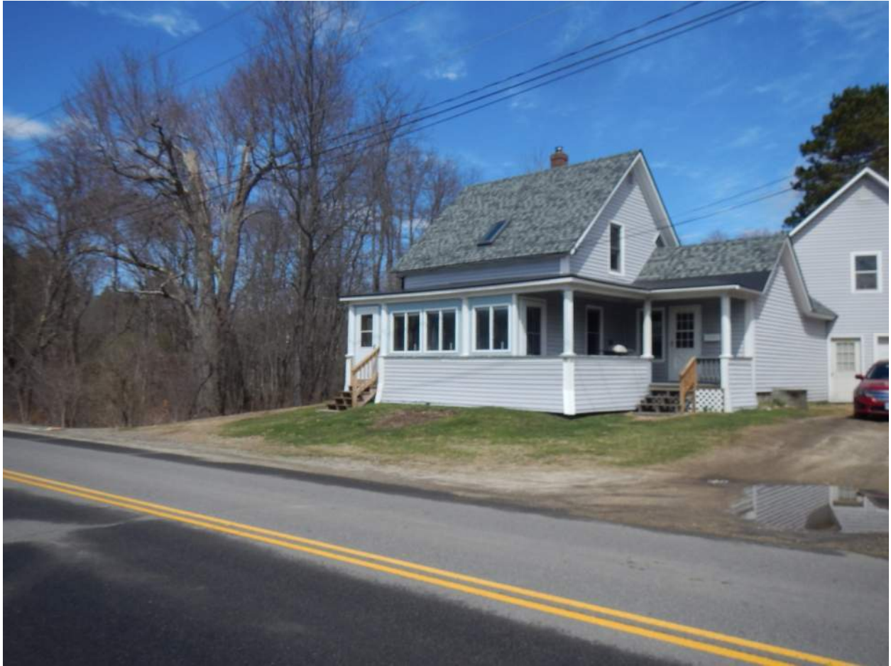
House at NE quadrant where guardrail will be extended
