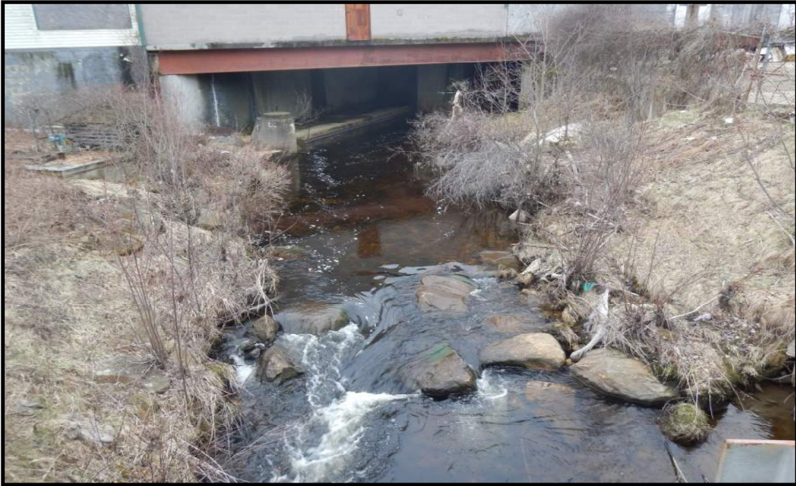
Photo 1: Outlet looking upstream
