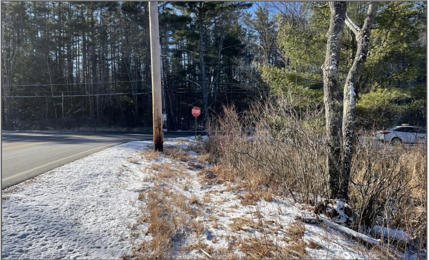
Photo 9: 15" Pipe Looking at Outlet Looking Southwest
