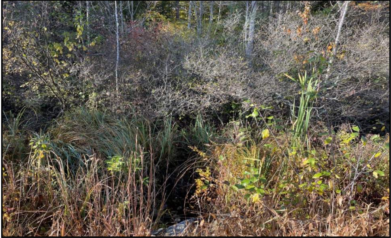
Photo 1: Inlet area for eastern most pipe (looking Northeast).
