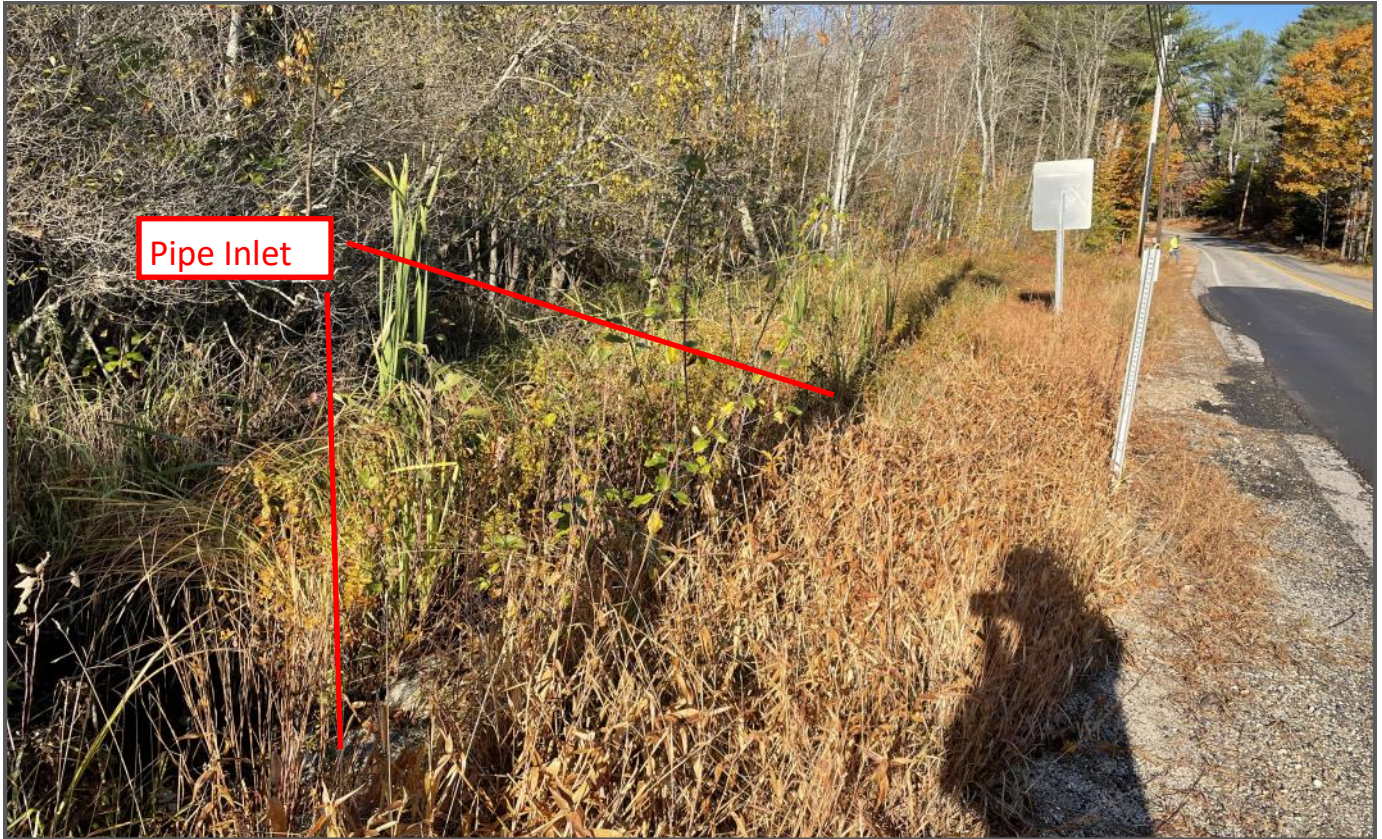
Photo 3: South Side of NH 109-A
