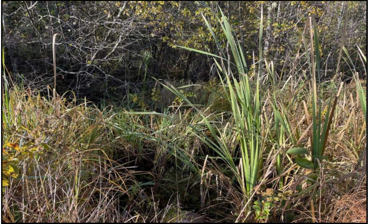
Photo 3: Inlet area of western most pipe (looking Northeast).
