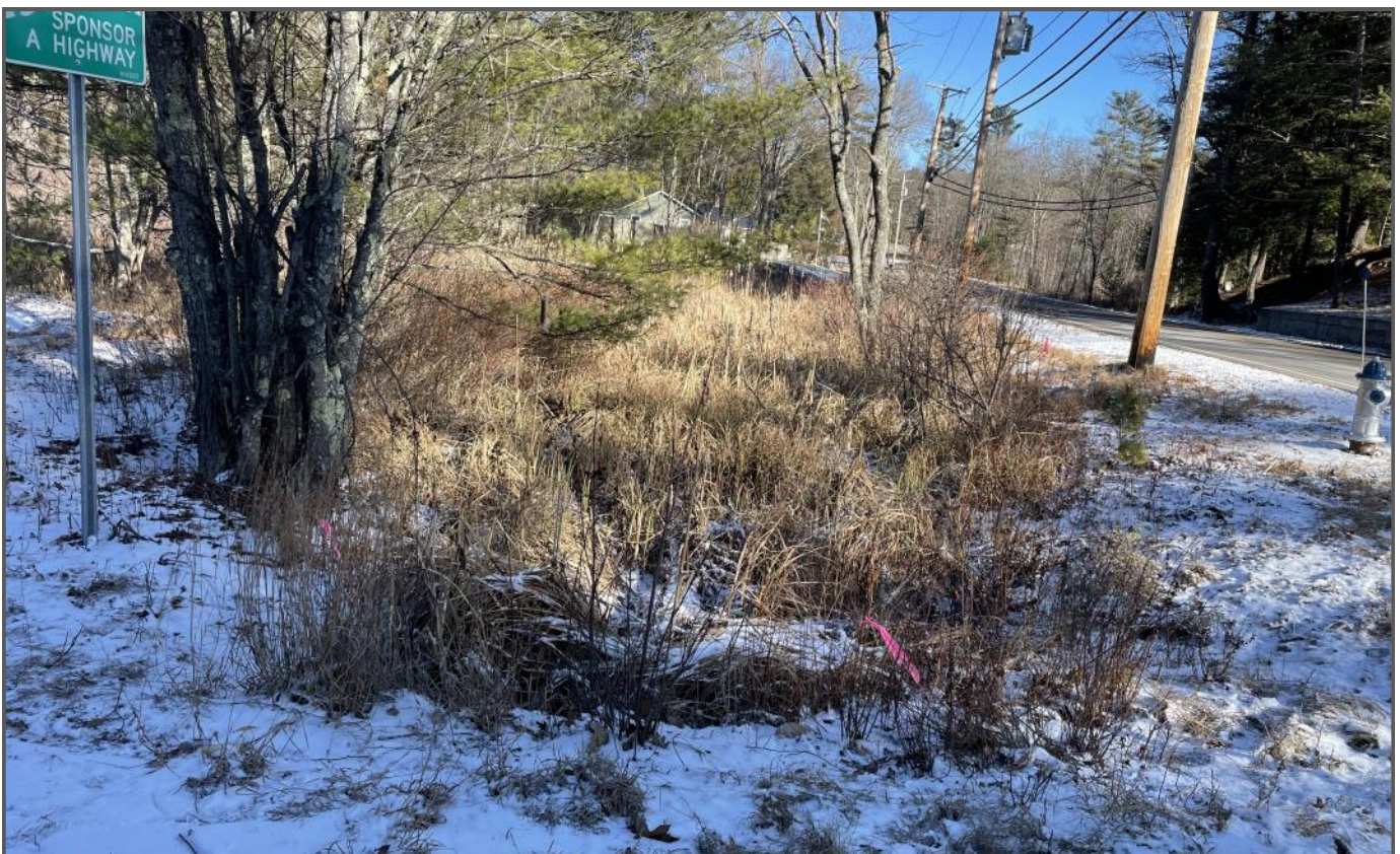
Photo 10: 15" Pipe from Outlet Looking Northeast
