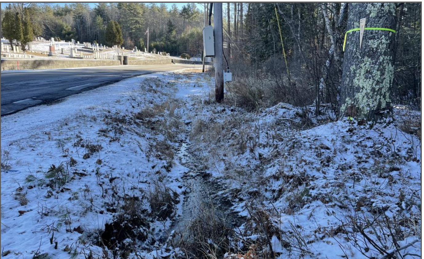
Photo 12: 15" Pipe from Inlet Looking Southeast
