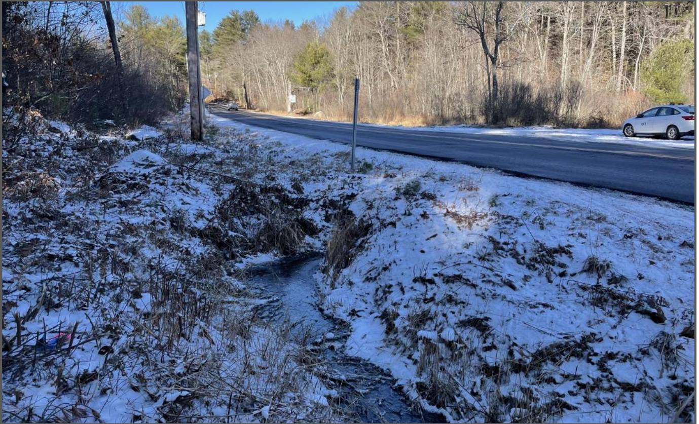
Photo 11: 15" Pipe at Inlet Looking Northwest
