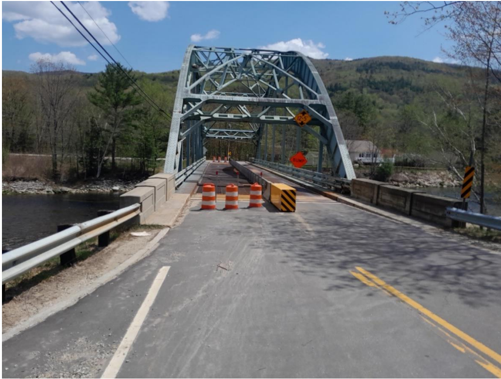
Photo 3: Facing east from west approach (5/11/2023)
