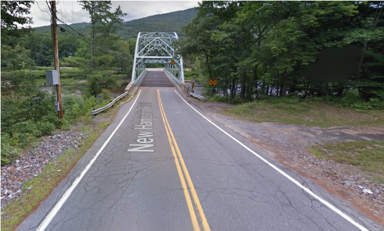
Photo 11: At western limit of project facing east toward impact areas A, B, and C (Google Maps image, 2014)
