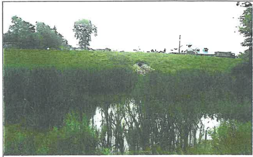
Photo 8. Wet detention basin constructed on parcel R5/Lot 20 looking east towards NH 125 and Landscapers Depot.
