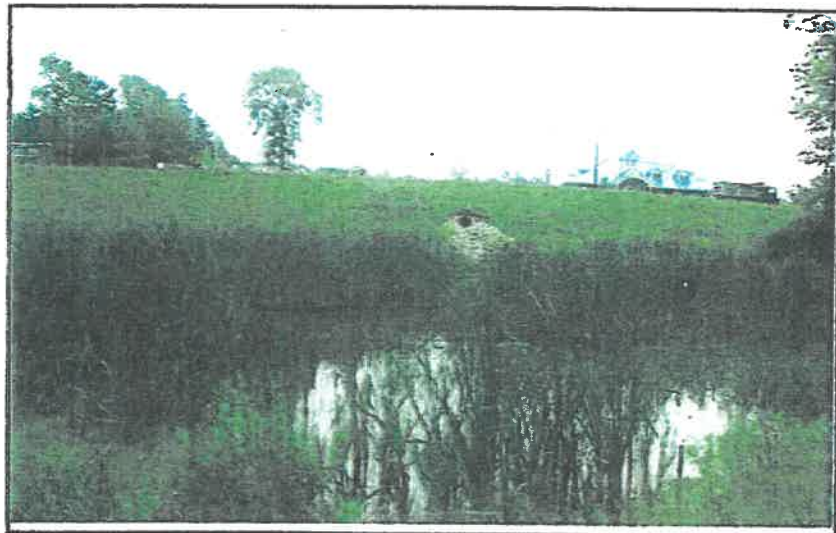
Photo 8. Wet detention basin constructed on parcel R5/Lot 20 looking east towards NH 125 and Landscapers Depot.
