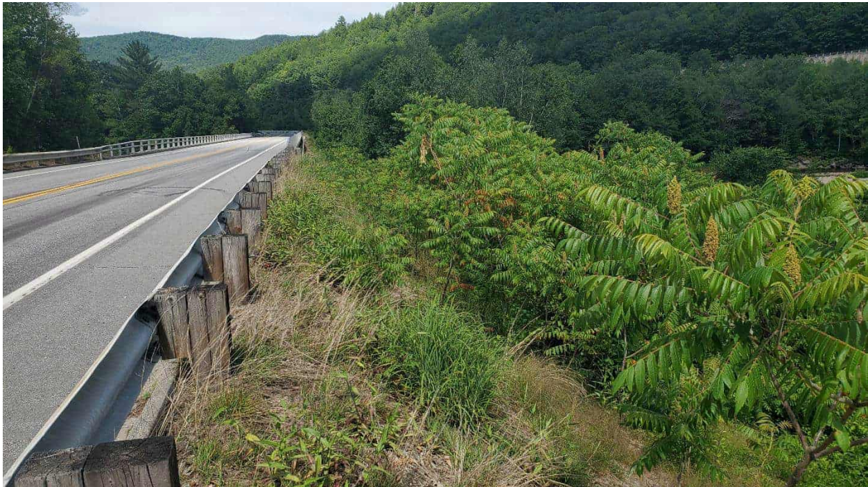
Figure 4. View of Route 175 (left side of photo) and slope where the temporary access road will be constructed to reach Pier 1 (looking northeast toward the bridge).
