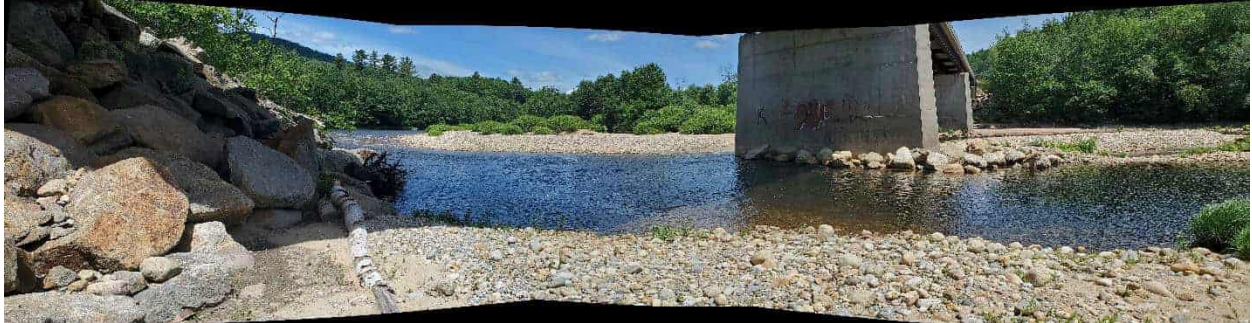
Figure 3. Panoramic view looking under the bridge in the project area at Pier 1 where the proposed causeway will be located (looking north).
