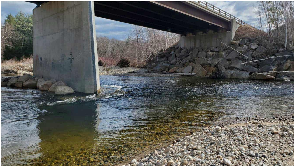
Figure 2. View of Pier I (the subject of this scour repair project). View is looking south.
