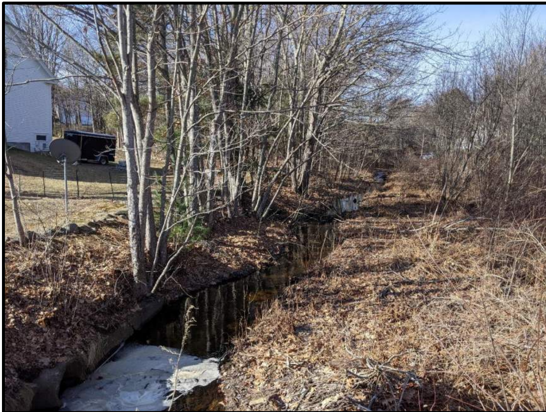
Photo 7: Upstream of Culvert Inlet (1/19/2021)
