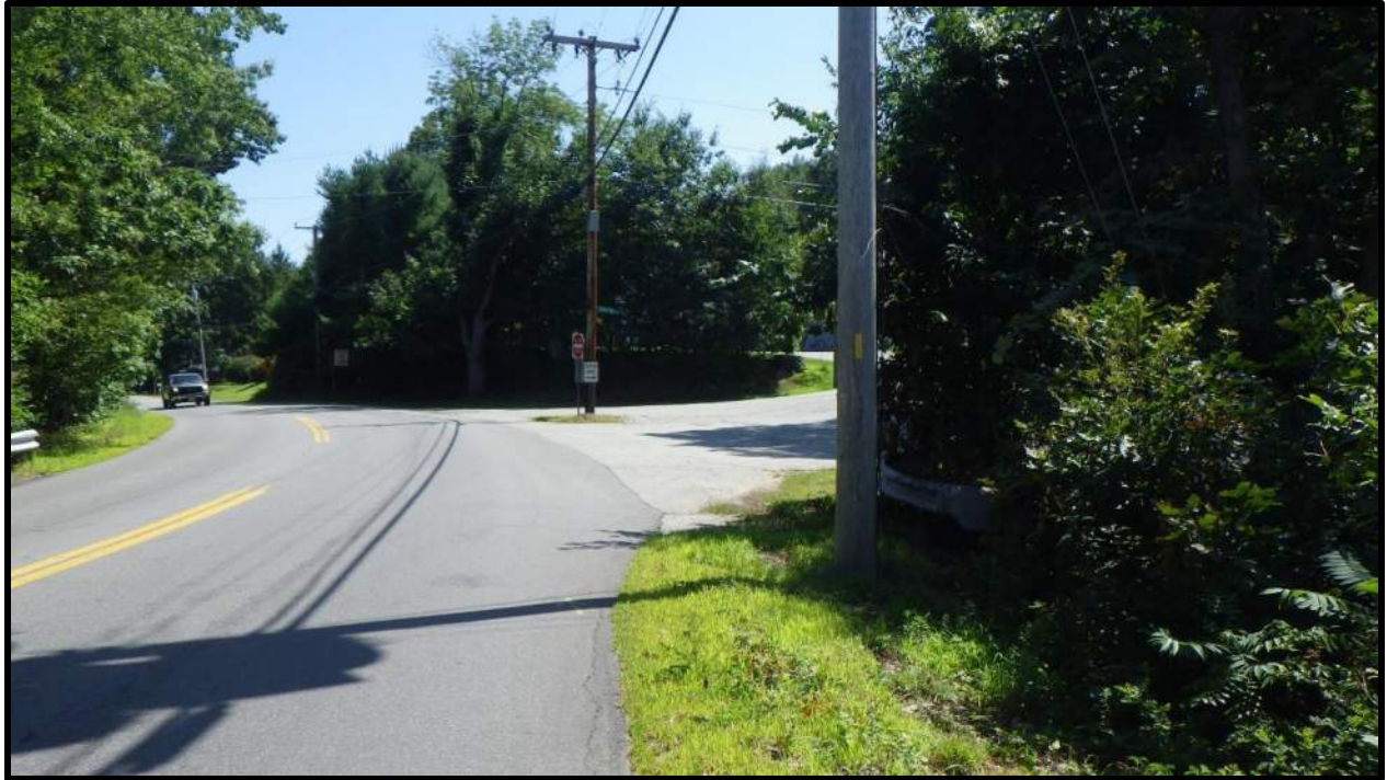
Photo 10: Amesbury Rd. Southerly Facing Goulds Hill Rd. (8/15/2019)
