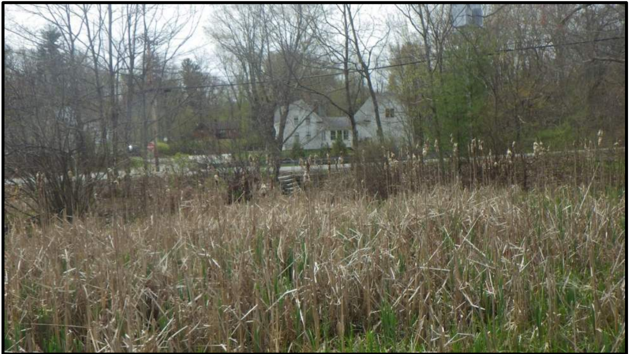
Photo 4: Culvert Outlet from Wetlands (5/6/2022)
