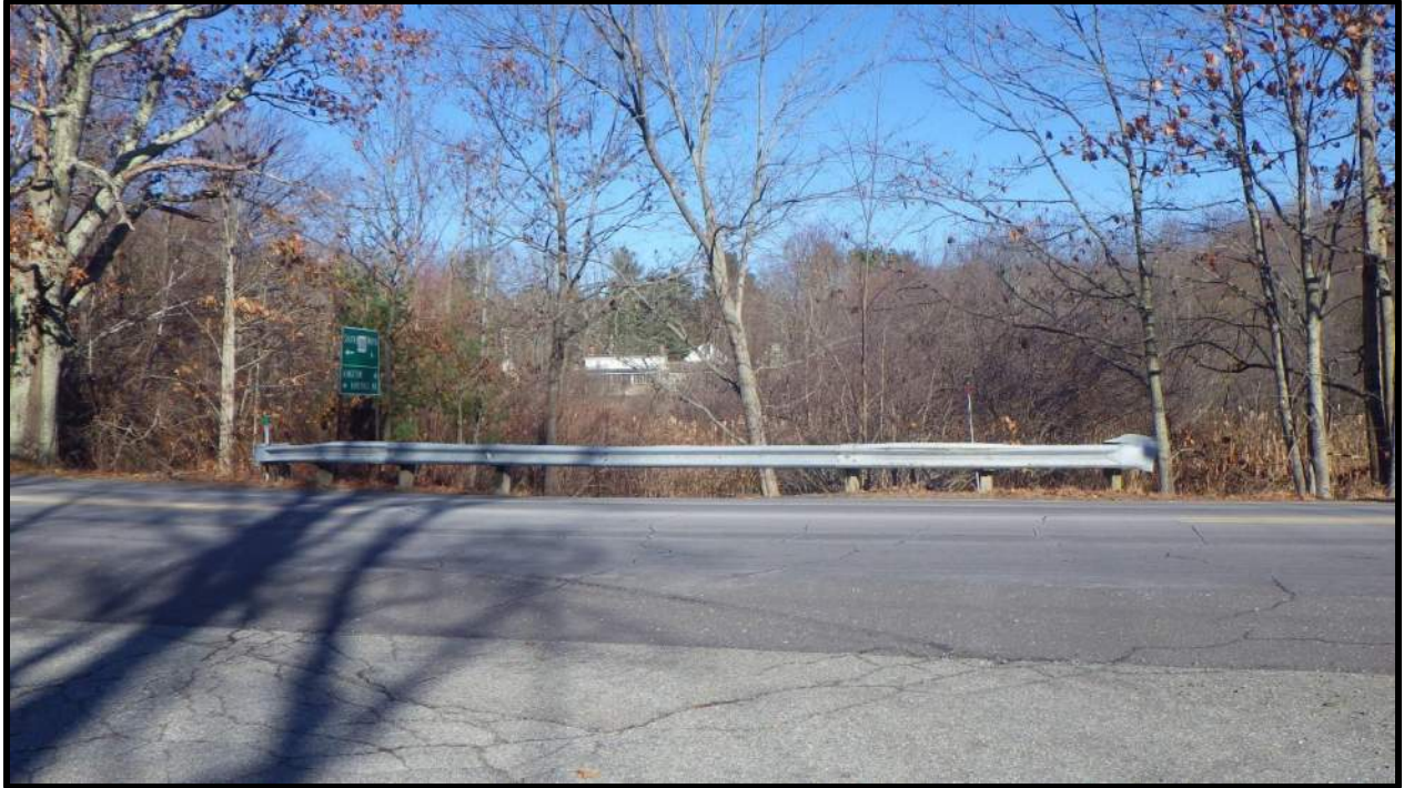
Photo 3: Culvert Outlet from Amesbury Rd. (11/21/2019)
