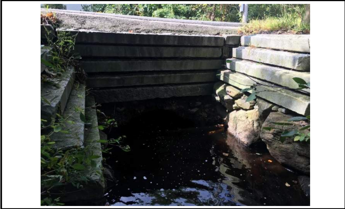
Photo 1: View of Outlet – Looking upstream
