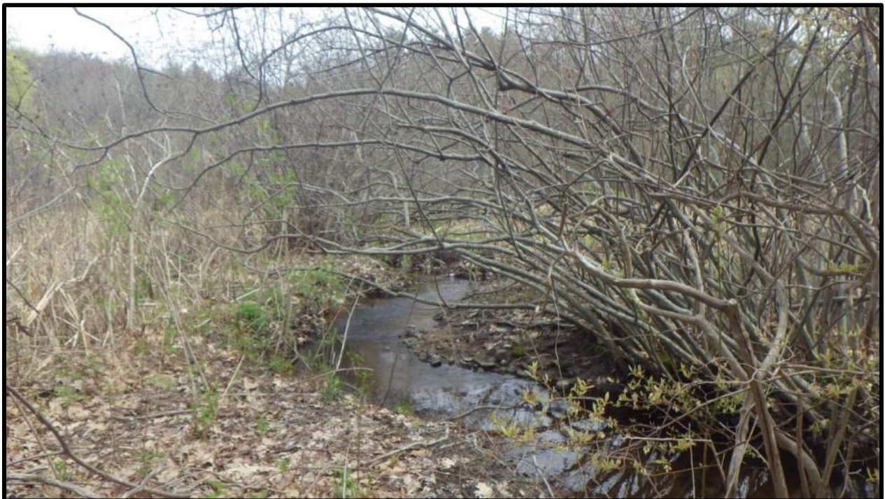
Photo 2: Wetlands Downstream of Culvert Outlet (5/6/2022)
