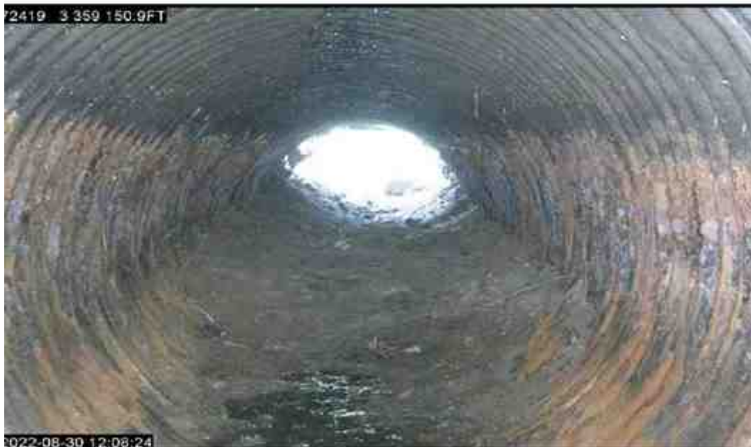
30" cmp - outlet inside
