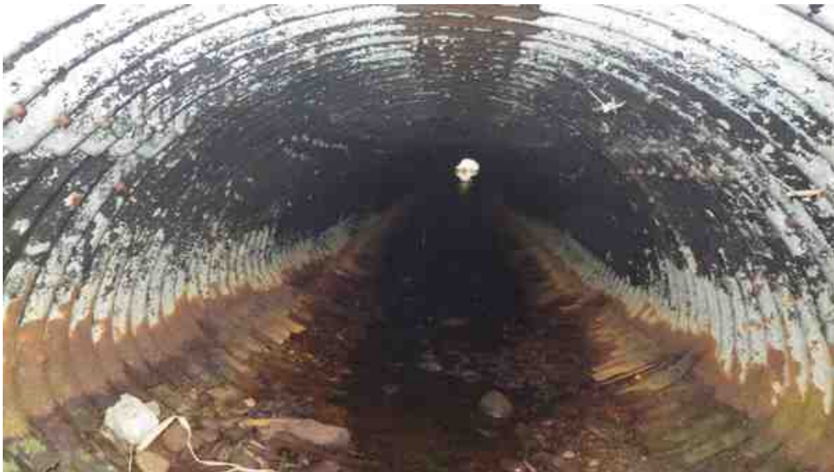
Location 3, 43" x 27" Culvert inside, showing heavy rust and invert deterioration
