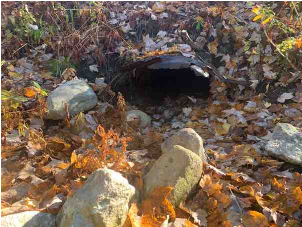
Location 1, 30" Culvert outlet, area of proposed stone apron Wetland #2 (PEM1E) - Impact Area B
