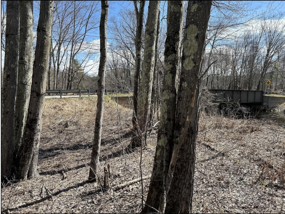
Photo 4. View east from the southwest bridge quadrant. Photo taken on 4/15/2024.
