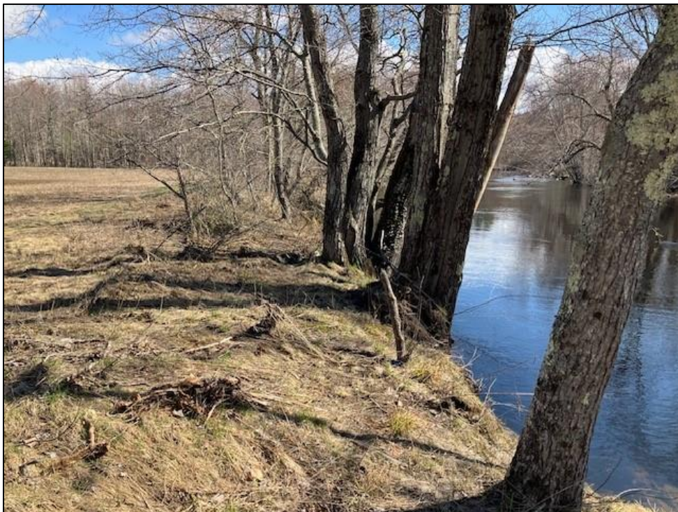
Photo 2. Blackwater River and bank in the northwest bridge quadrant, view northeast. Photo taken on 4/15/2024.
