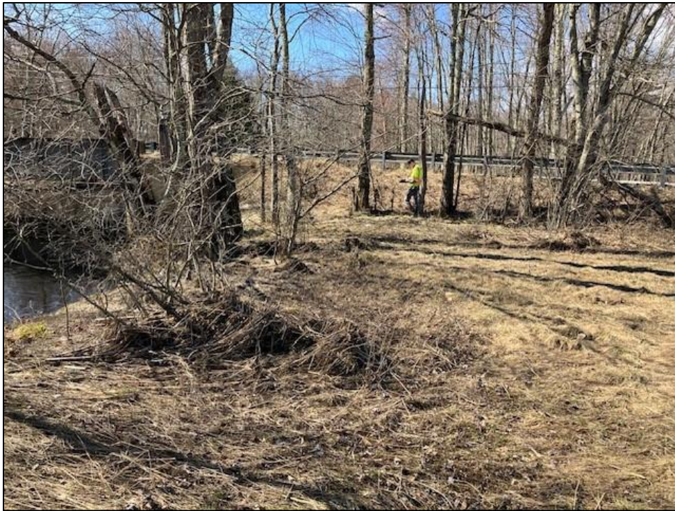
Photo 1. View southwest toward US Route 4 from the northwest bridge quadrant. Photo taken on 4/15/2024.
