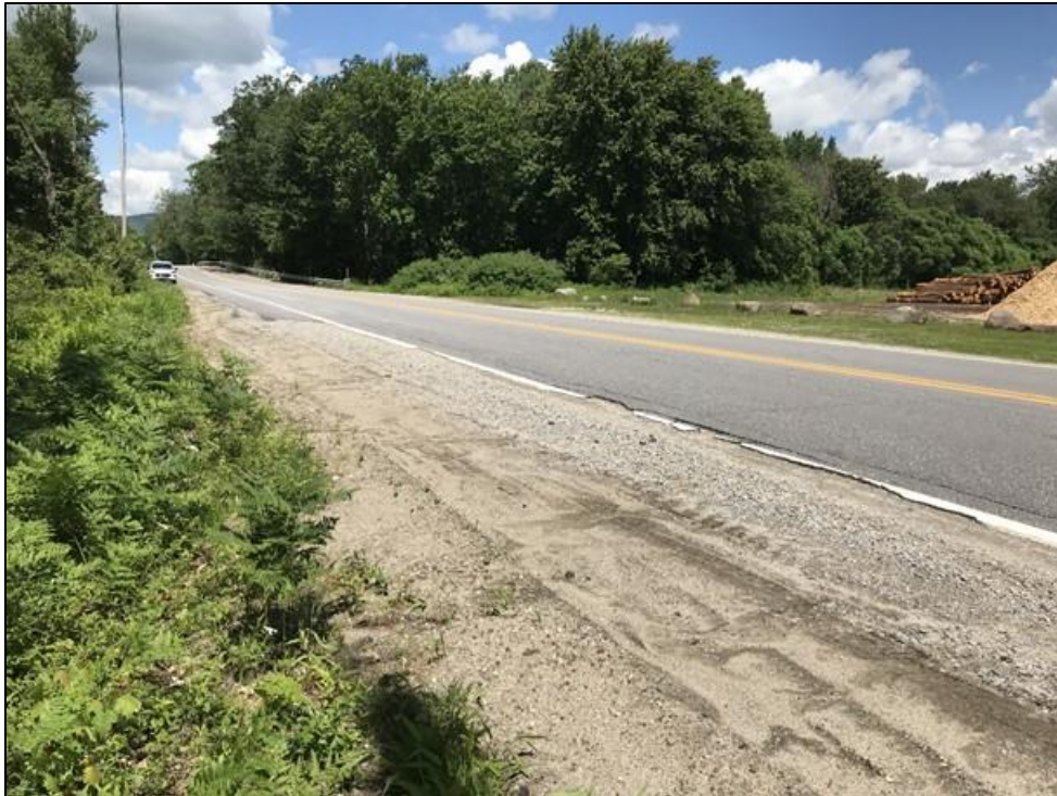
Photo 9. View northwest toward Bridge No. 143/077. Photo taken on 6/10/2022.
