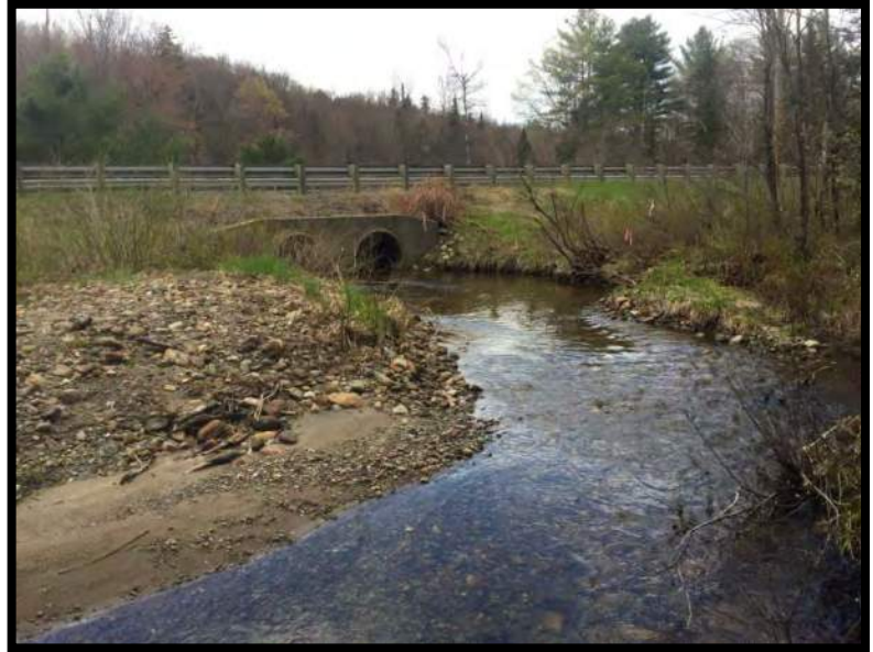
This is a view of the crossing structure looking upstream.
