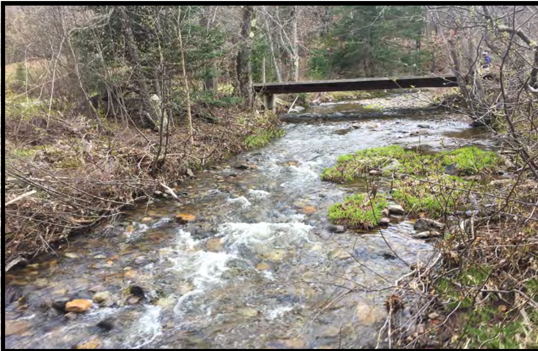
PHOTO 3: This is a view looking upstream away from the crossing at site 1.
