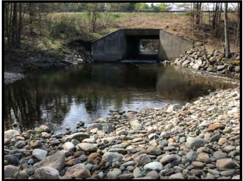
This is a view looking upstream towards the crossing structure.
