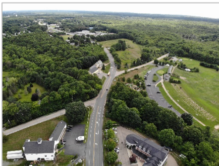
Route 1 Reconstruction & North Road Realignment | North Hampton
