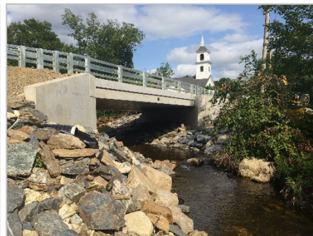
Route 123A over Bowers Brook Bridge Replacement | Acworth
