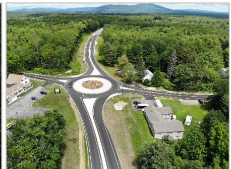
Route 28 & Route 171 Roundabout | Ossipee
