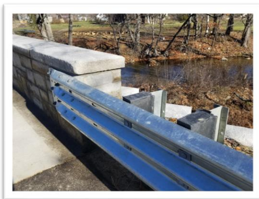
Connection Plate and Thrie-Beam Terminal Connector
