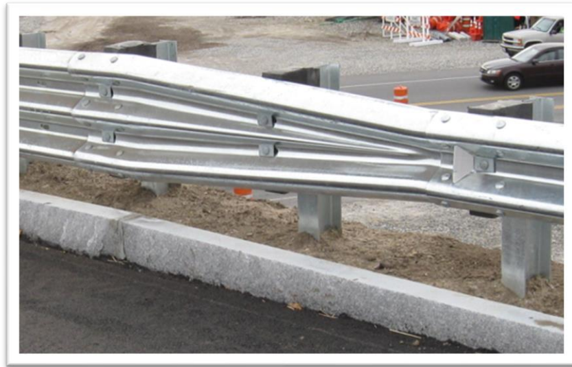
Thrie-Beam Transition Rail Section
