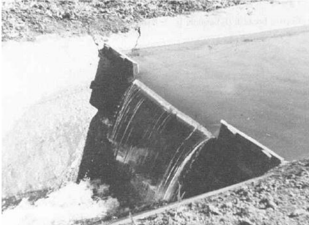
Figure 4.0.13.c Sharp crested weir
