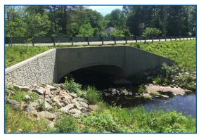
Buried structures provide an economical, environmentally friendly, and low maintenance solution for many small bridges.
