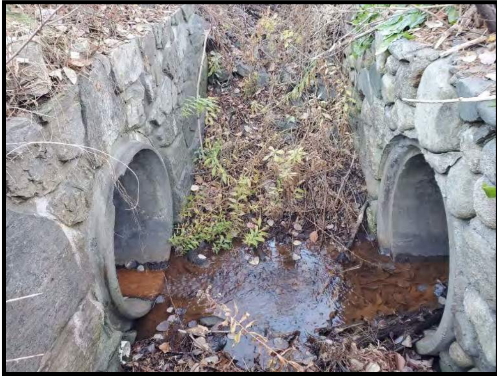
Photo 15 – Stream 3 View of Two Headwalls Facing East – 11/3/2022
