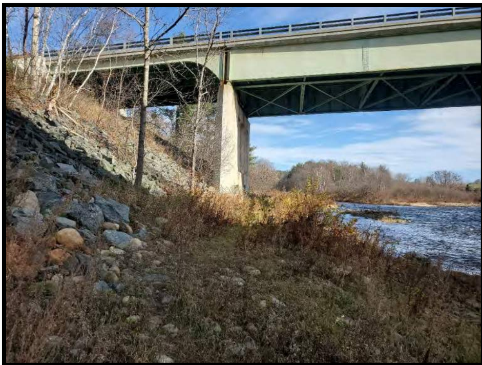
Photo 2 – Ammonoosuc North Bank Under Southbound Bridge Facing Upstream/NE – 11/2/2022
