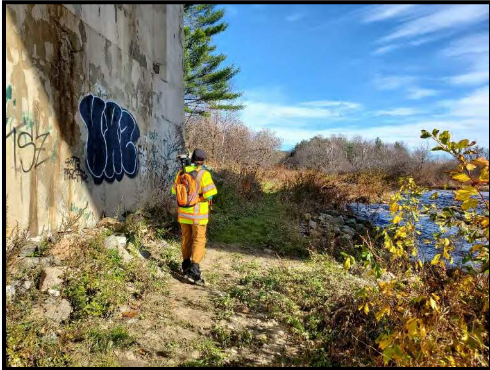
Photo 3 – Ammonoosuc North Bank Under Northbound Bridge Facing Upstream/NE – 11/2/2022
