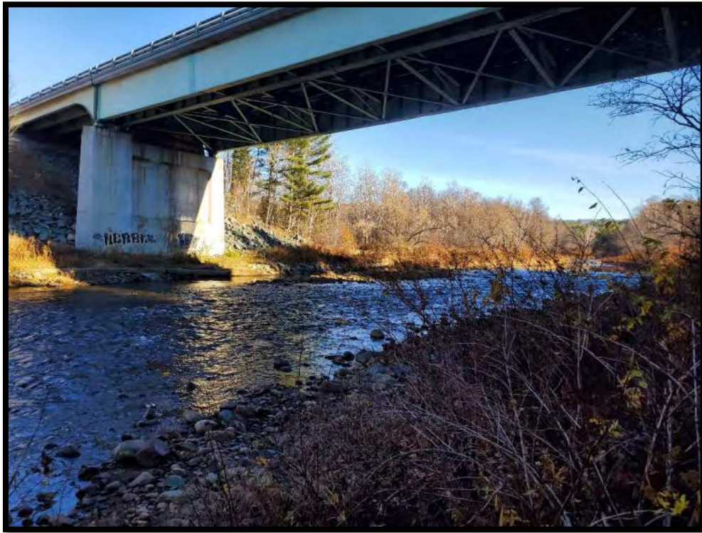
Photo 17– Ammonoosuc South Bank Between NB and SB Bridges Facing Northeast – 11/3/2022
