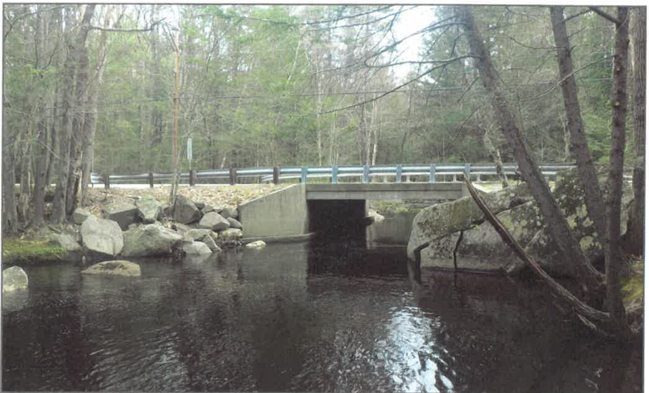
Photo 4: Looking East (downstream) at bridge inlet
