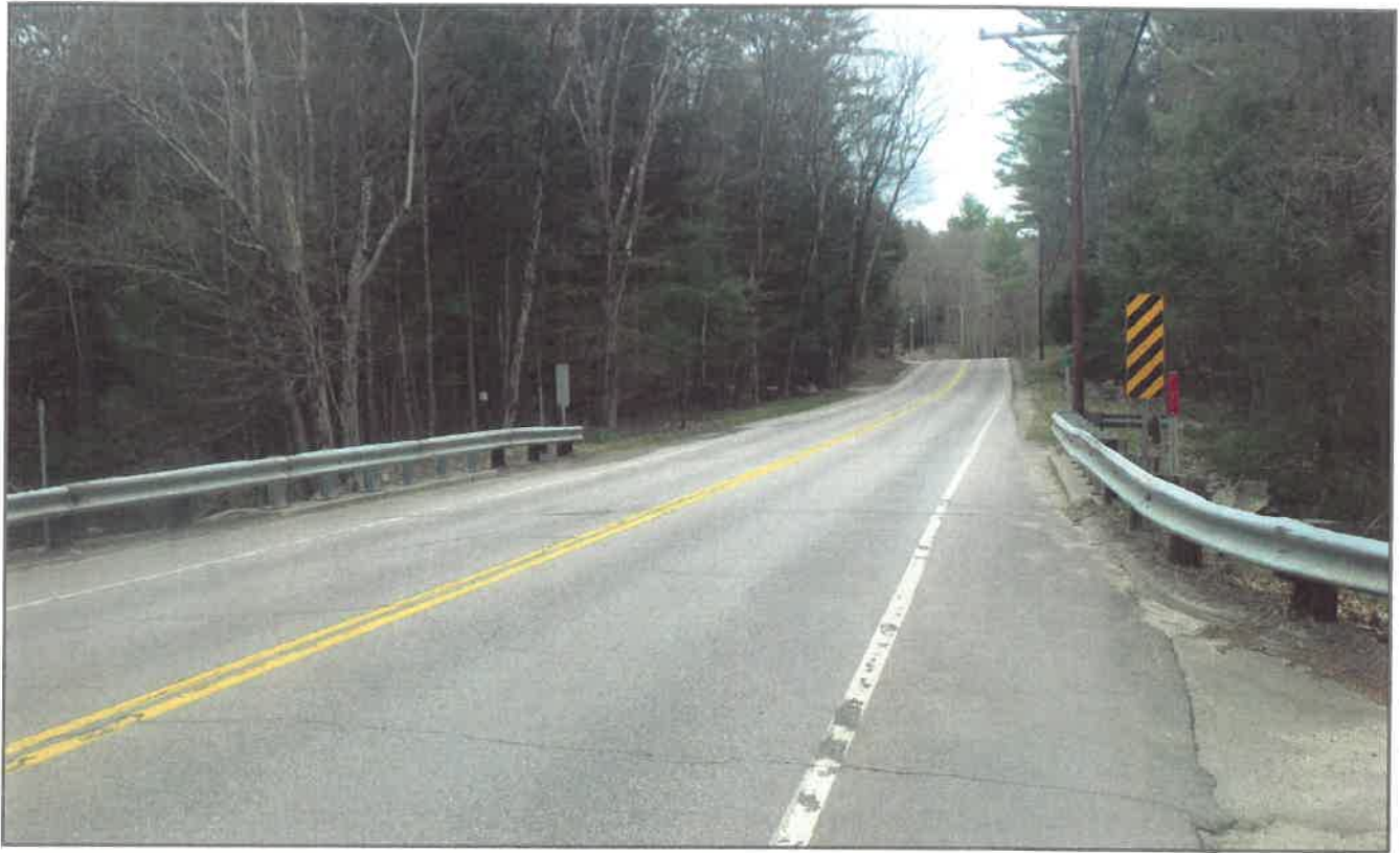
Photo 1: Looking South along NH 31, toward Lyndeborough
