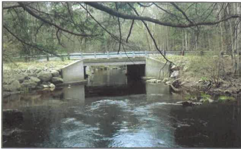
Photo 6: Looking West (upstream) at bridge outlet
