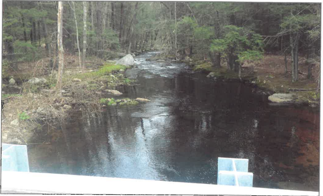
Photo 5: Looking East (downstream) from NH 31
