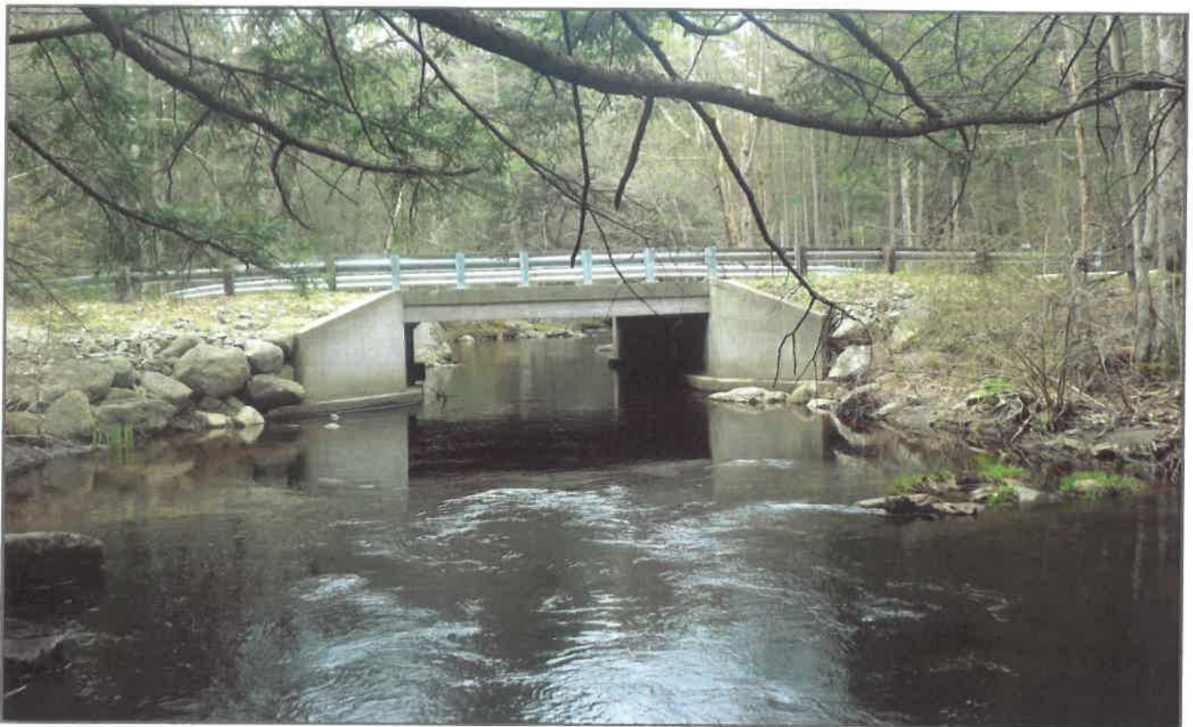
Photo 6: Looking West (upstream) at bridge outlet
