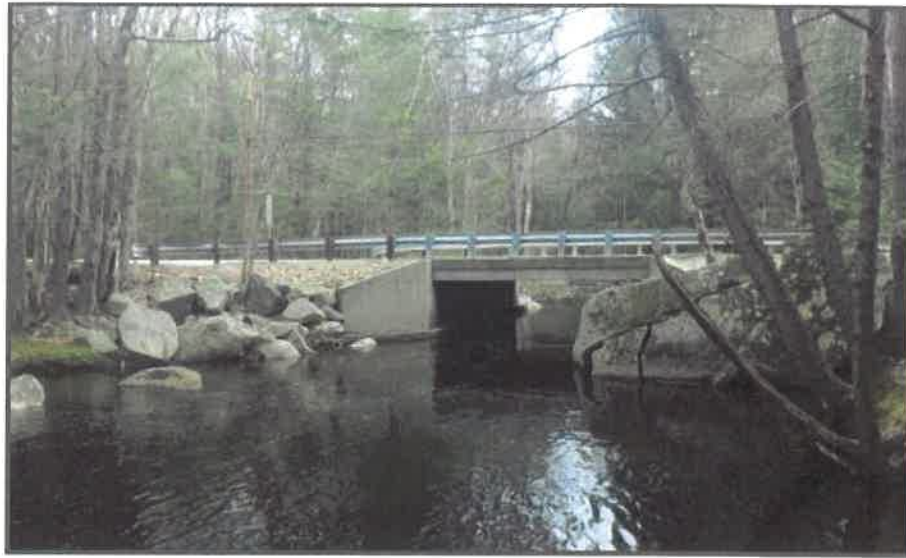
Photo 4: Looking East (downstream) at bridge inlet
