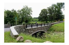
bridge, special care was taken in selecting the aesthetic treatments including a stone form liner, painted bridge rail, and timber guiderail on the approaches.
