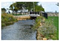
Replacement of Town Brook Bridges - Plymouth, MA: The Town of Plymouth retained SLR to design the removal of several dams and outlet structures and replacement with three bridges. This work, along with the design of channel modifications, allowed restoration of herring migration through this section of
