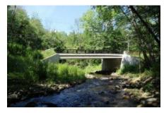
along each fascia. The bridge superstructure is supported on concrete abutments. The firm provided survey; hydrologic, hydraulic, and scour analysis; wetland delineation; permitting; and roadway engineering and structural engineering services.
