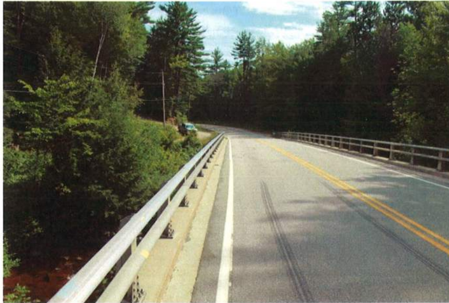
Photo 1: View south over bridge, NH Route 113A. 8/22/19
