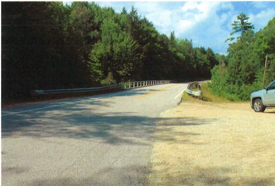
Photo 2: View north over bridge, NH Route 113A. 8/22/19
