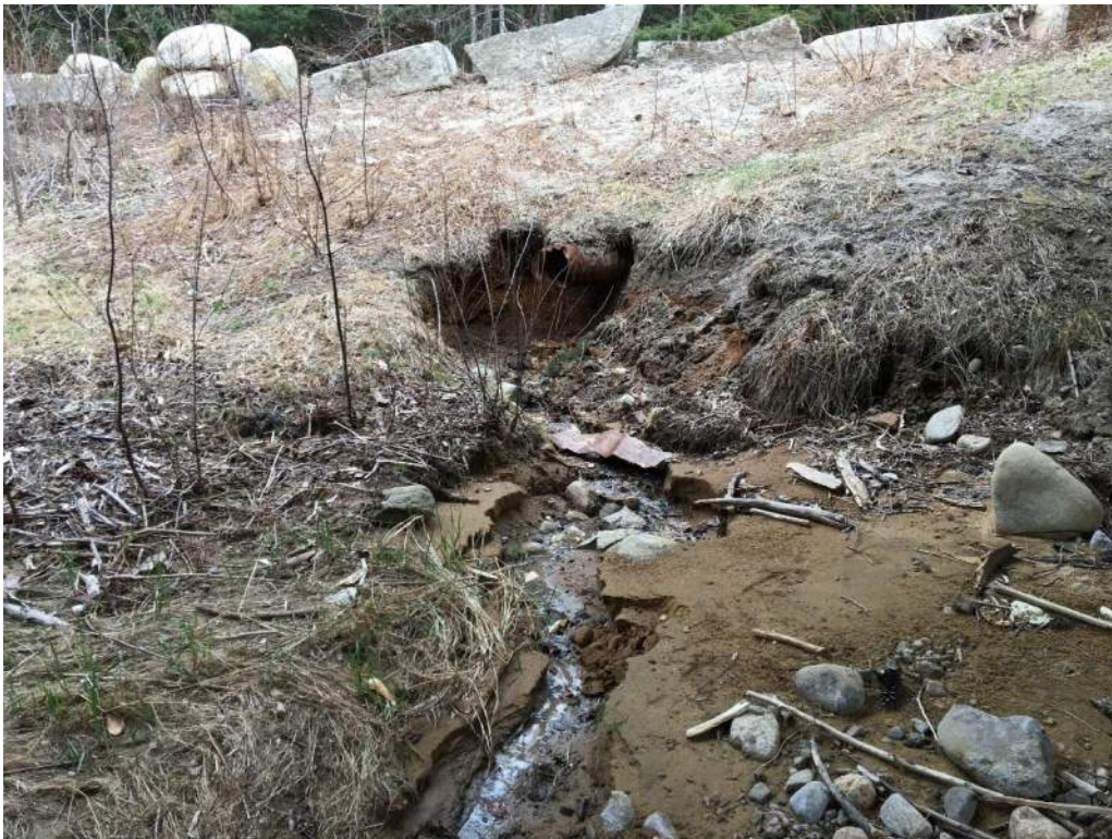
Photo 9: IMPACT AREAS: A & E – Bank behind southern bridge pier showing erosion/scour from existing drainage outfall (05/06/2020) Photo Direction: SE
