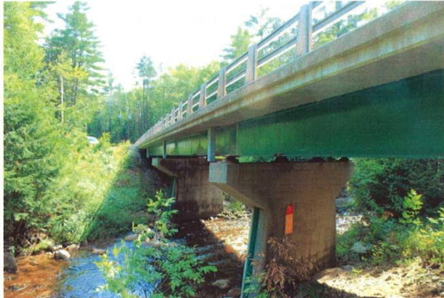
Photo 3: Eastern elevation of Bridge #061/091, NH Route 113A. 8/22/19
