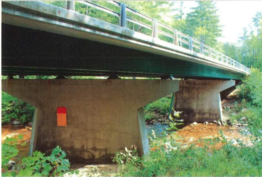
Photo 5: Western elevation of Bridge #061/091. 4/25/19
