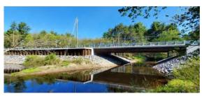
Bedford Road experienced frequent roadway over topping. Based on hydraulic requirements, TTG designed a replacement structure that utilized a 90-foot span plate girder, concrete bridge deck, founded on steel piles with cast-inplace concrete pile caps.
