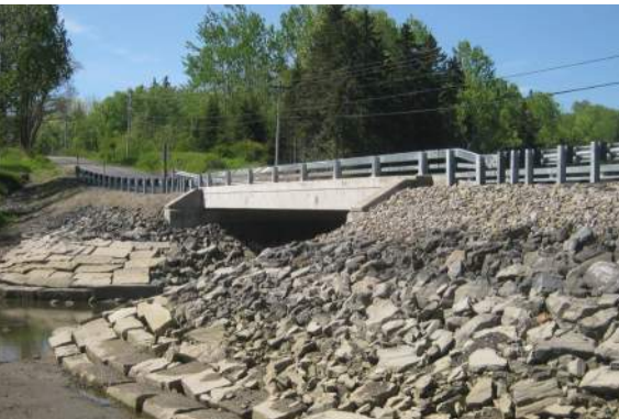
Mill Bridge over Mill Creek
