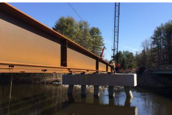
Covered Bridge over Little Androscoggin River
