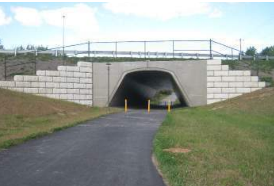
I-395 over Webster Avenue Pedestrian Tunnel
