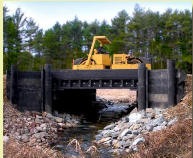
Birch Hill Road Culvert Replacement York, Maine
