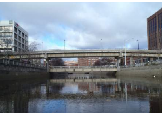
Kenduskeag Stream Pedestrian Bridge
