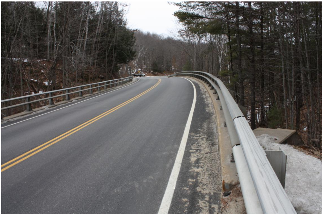
Photo # 13 Description: Roadway view Reference: 5514 Direction: east
