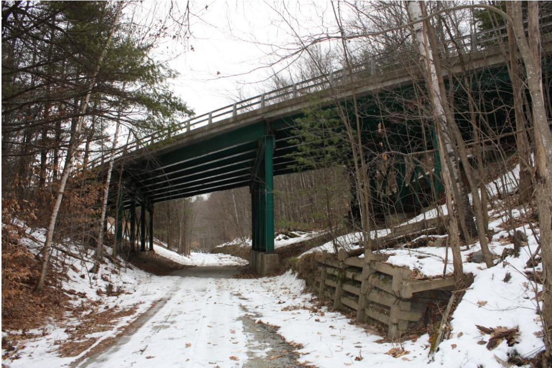
Photo # 2 Description: View down trail at north side of bridge with concrete tie crib wall at right Reference: 5479 Direction: SE
